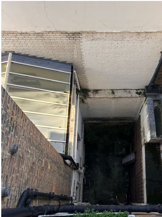
Photograph of Existing lightwell from 2 nd Floor
