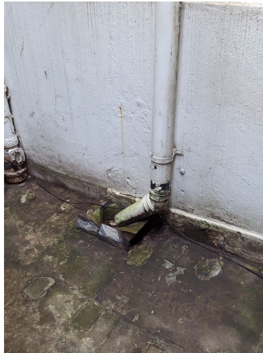
Photograph of Existing ground covering in lightwell
