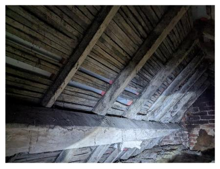
Internal photo of the front roof slope which shows the retention of the existing tiling lathes and original roof construction.
