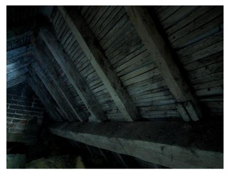
Internal photo of the rear roof slope which shows the retention of the existing tiling lathes and original roof construction.
