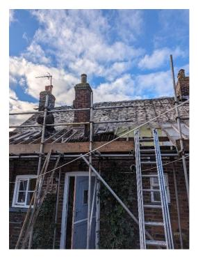
External appearance of the rear roof slope after stripping off roof tiles and roofing felt, to expose the existing pargetting and original tiling lathes, all of which have been retained during the course of the works.
