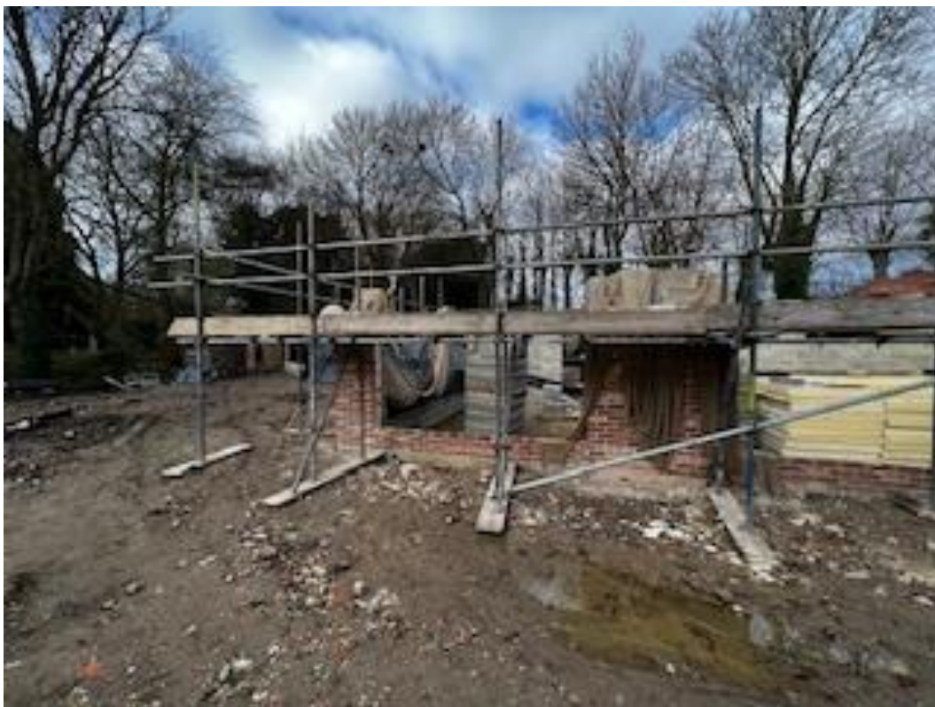
View looking north, with trees to Church Lane behind
