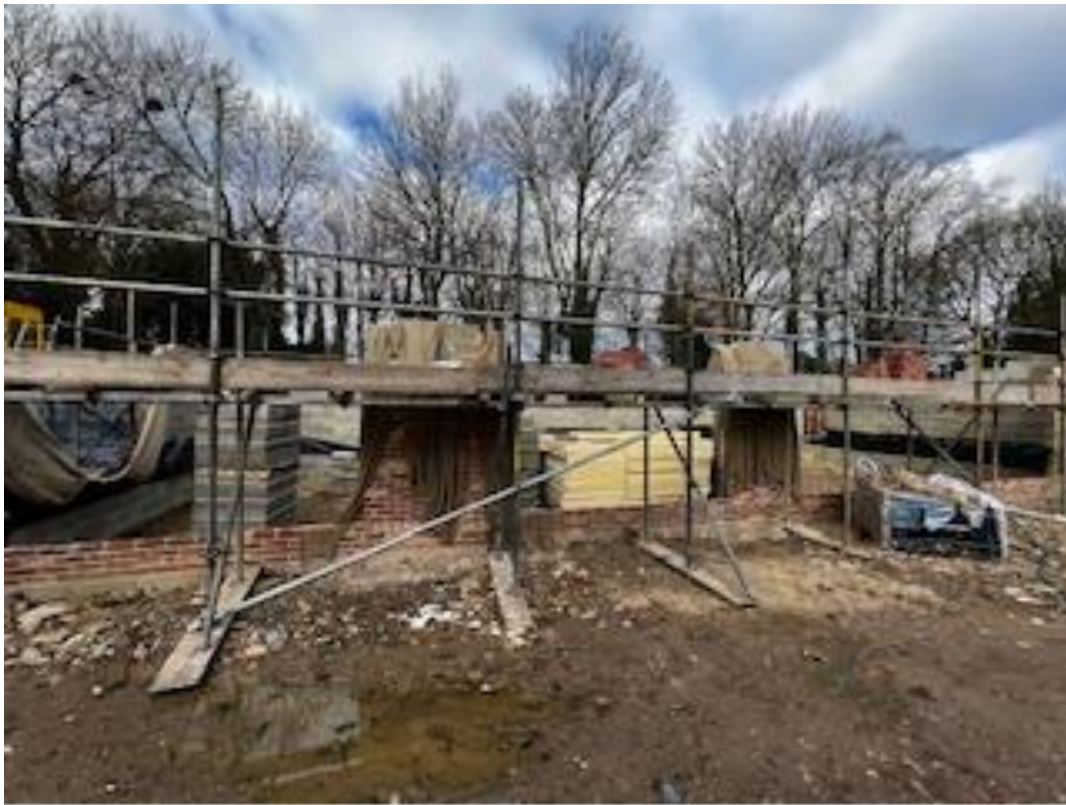
View looking north, towards Church Lane
