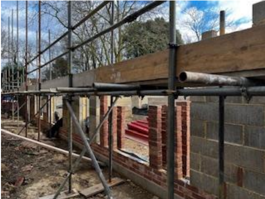
View of 'front' elevation, taken from north-west
