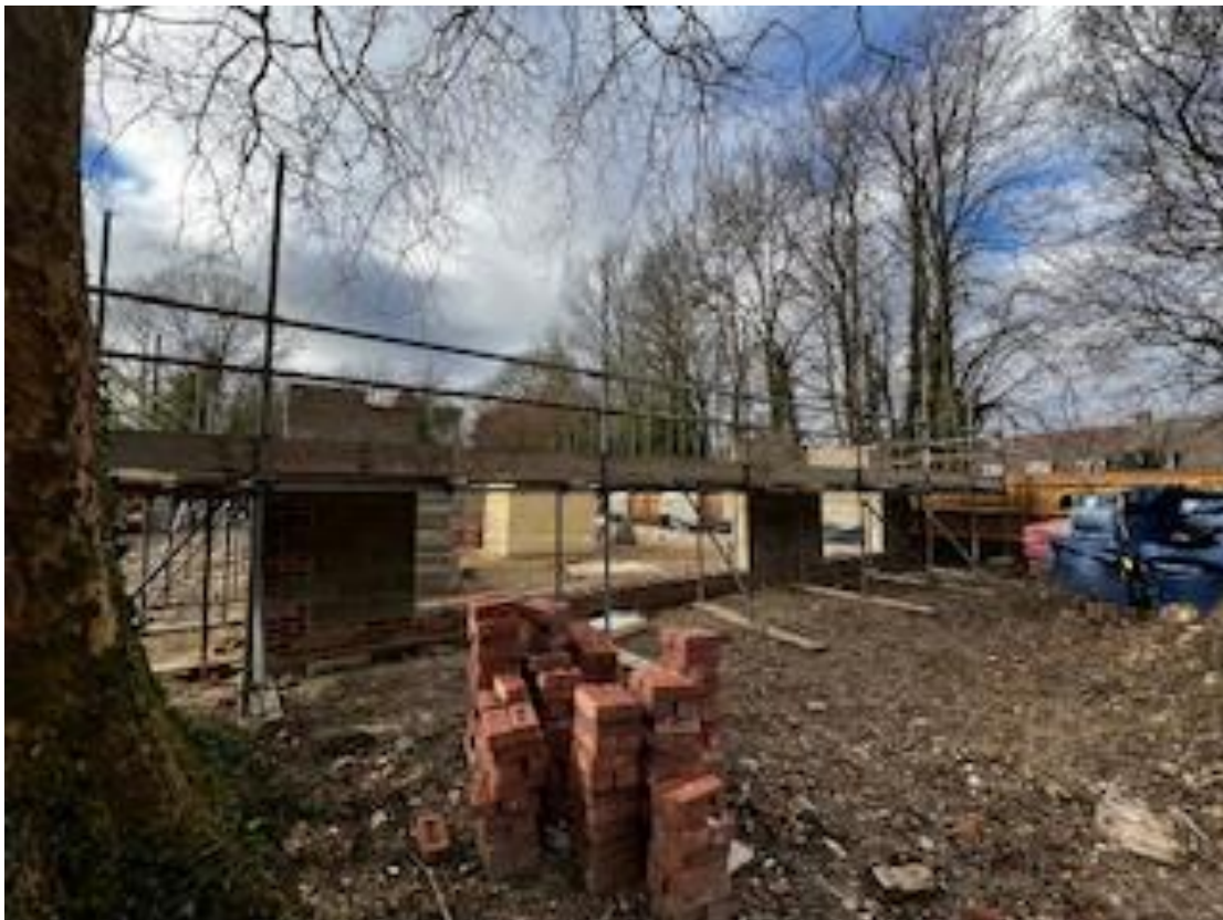
View from east, towards 'side' elevation
