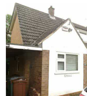
Picture showcasing existing extension to property
