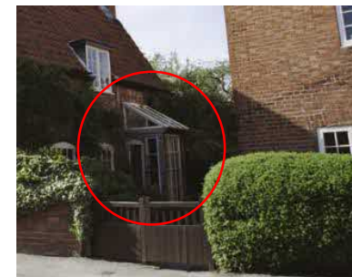
White framed porch with glazing
