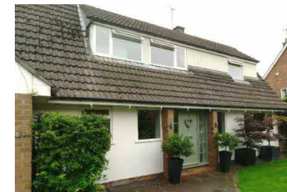
Unappealing front facade, not in-keeping with local character. Dormered windows, sloped roof, mismatched windows.
