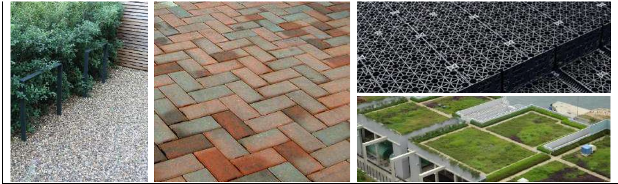
Figure 3: Surface water storage facilities and potential SuDS features - rainwater harvesting, on-site tank storage, rain garden soak-away and green roofs. (Source: UK SuDS Manual)
