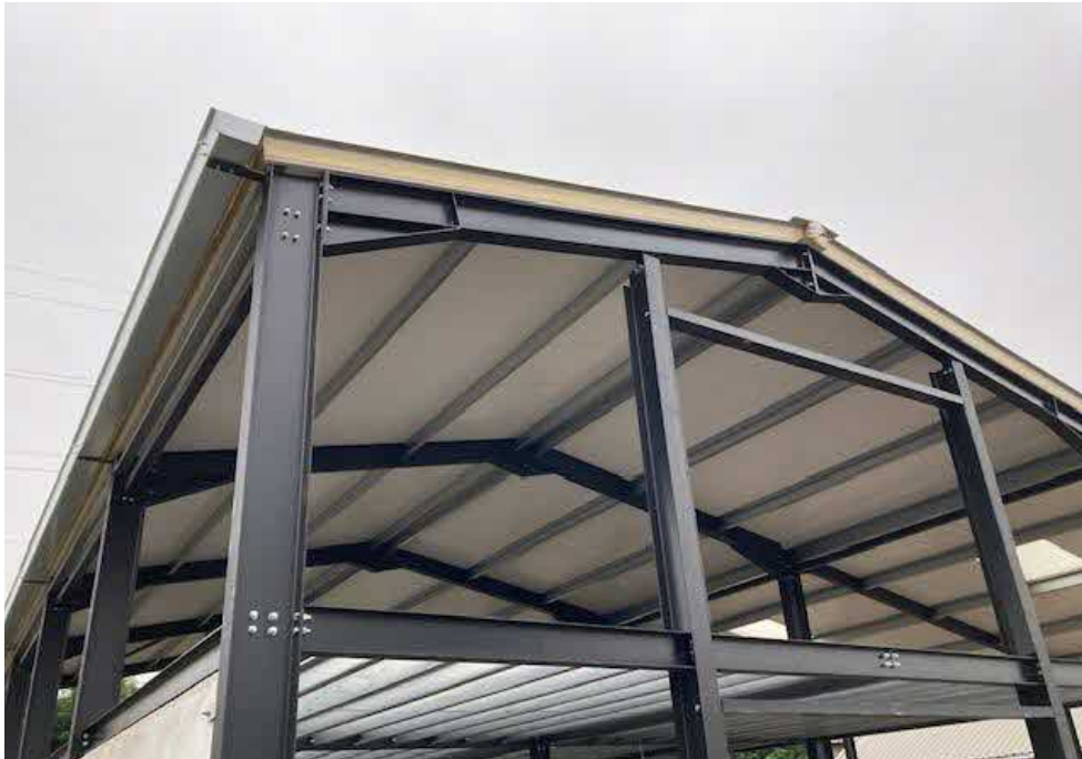
10. Steelwork, roof covering and galvanised box gutter at the front east corner.
