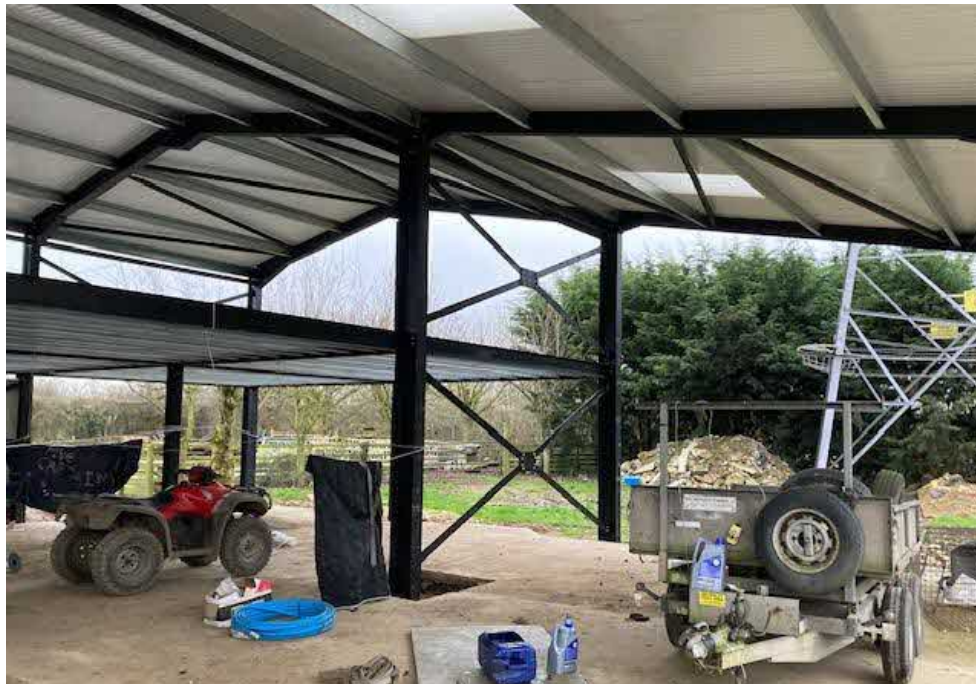
8. Looking through the building to the rear south corner.
