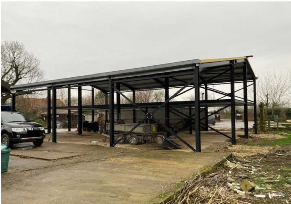
5. The rear west corner of the building.
