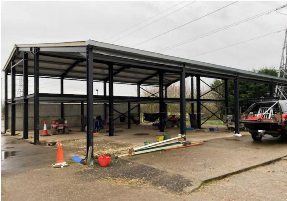
6. The front north corner of the building.
