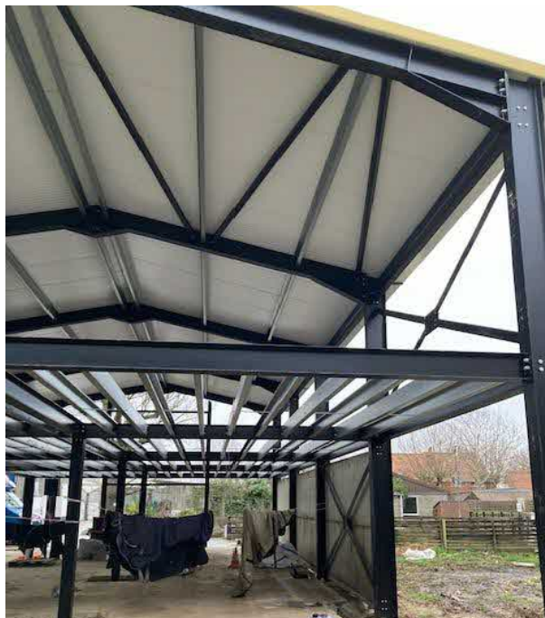
10. Steelwork, roof covering and galvanised box gutter at the front east corner.
