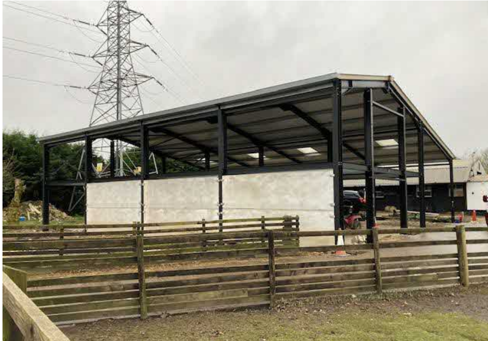
2. The front east corner of the new framed equestrian building.
