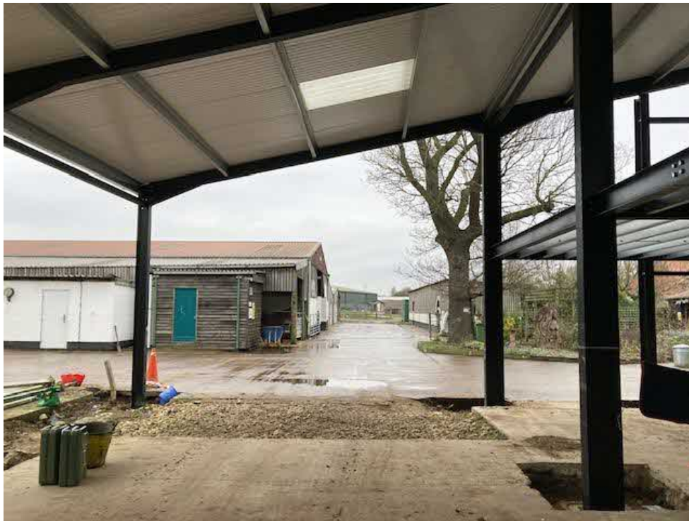
12. Looking out of the front north west side of the building.
