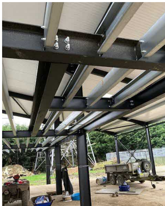
9. Steelwork in the centre of the building.
