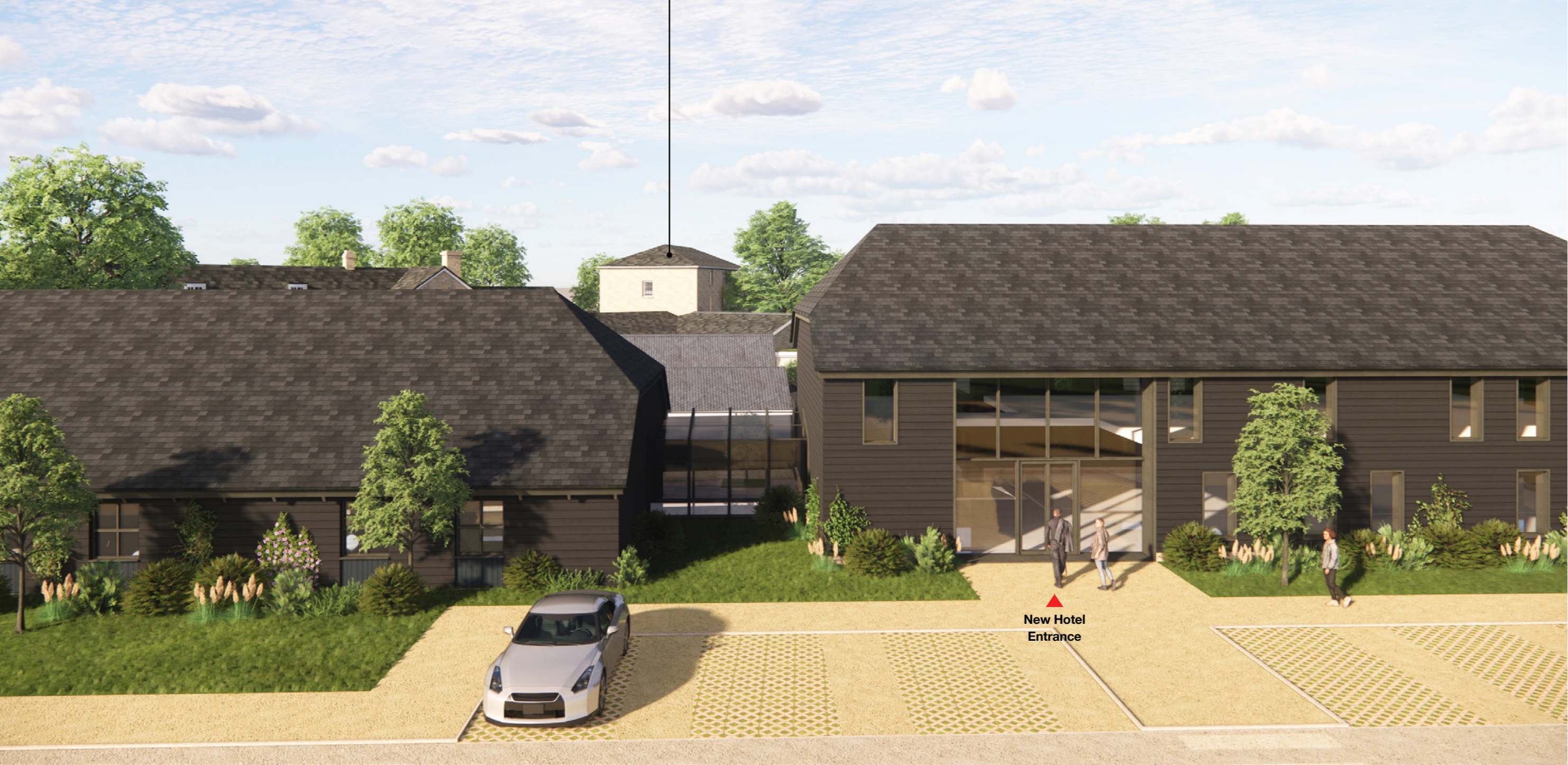
Quy Mill (Grade II listed)
