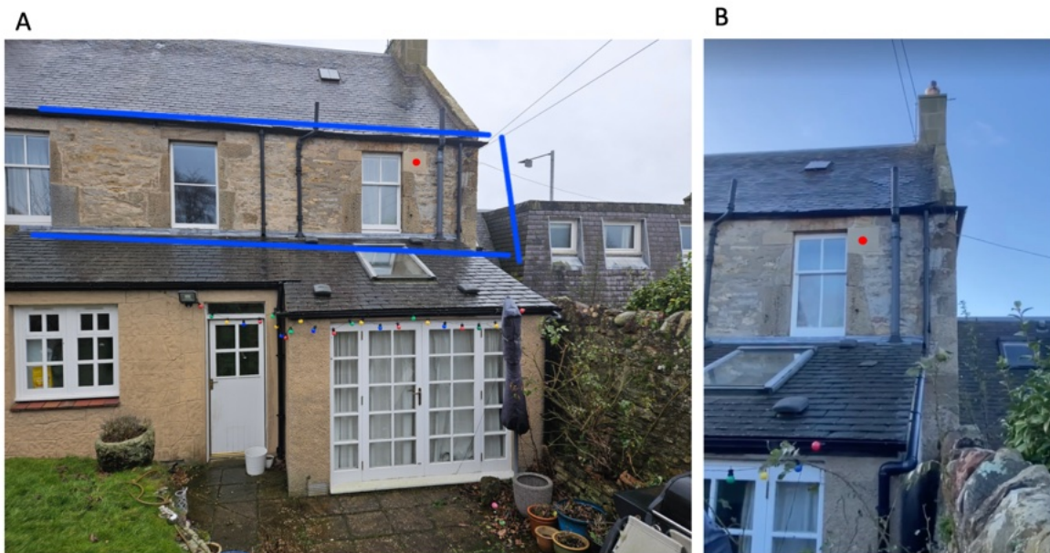
Figure 7: Position of the proposed vent in the rear elevation marked as red spots. The diameter will be 100 mm.
