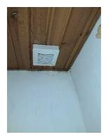
The dampness in this area as marked on the attached drawing would appear to be due to condensation caused by cold spotting within the Edinburgh Press cupboard and a lack of ventilation within the Bathroom on the Upper Floor.
