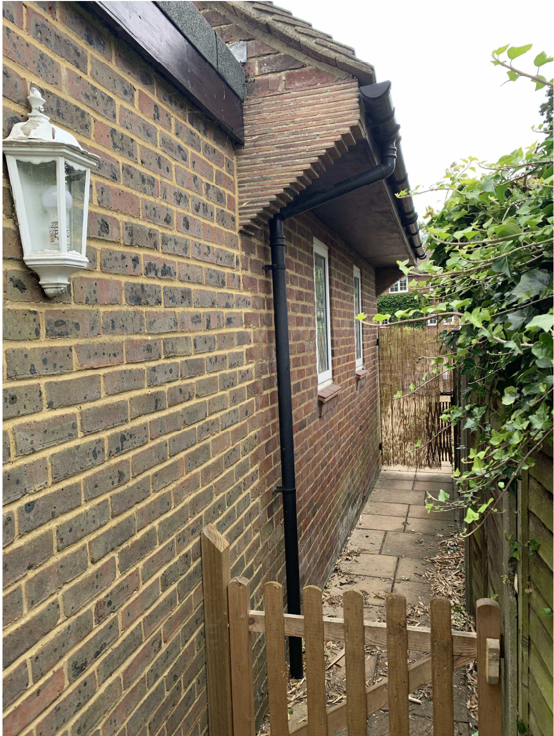
The side entrance giving access to the Dog Grooming Room
