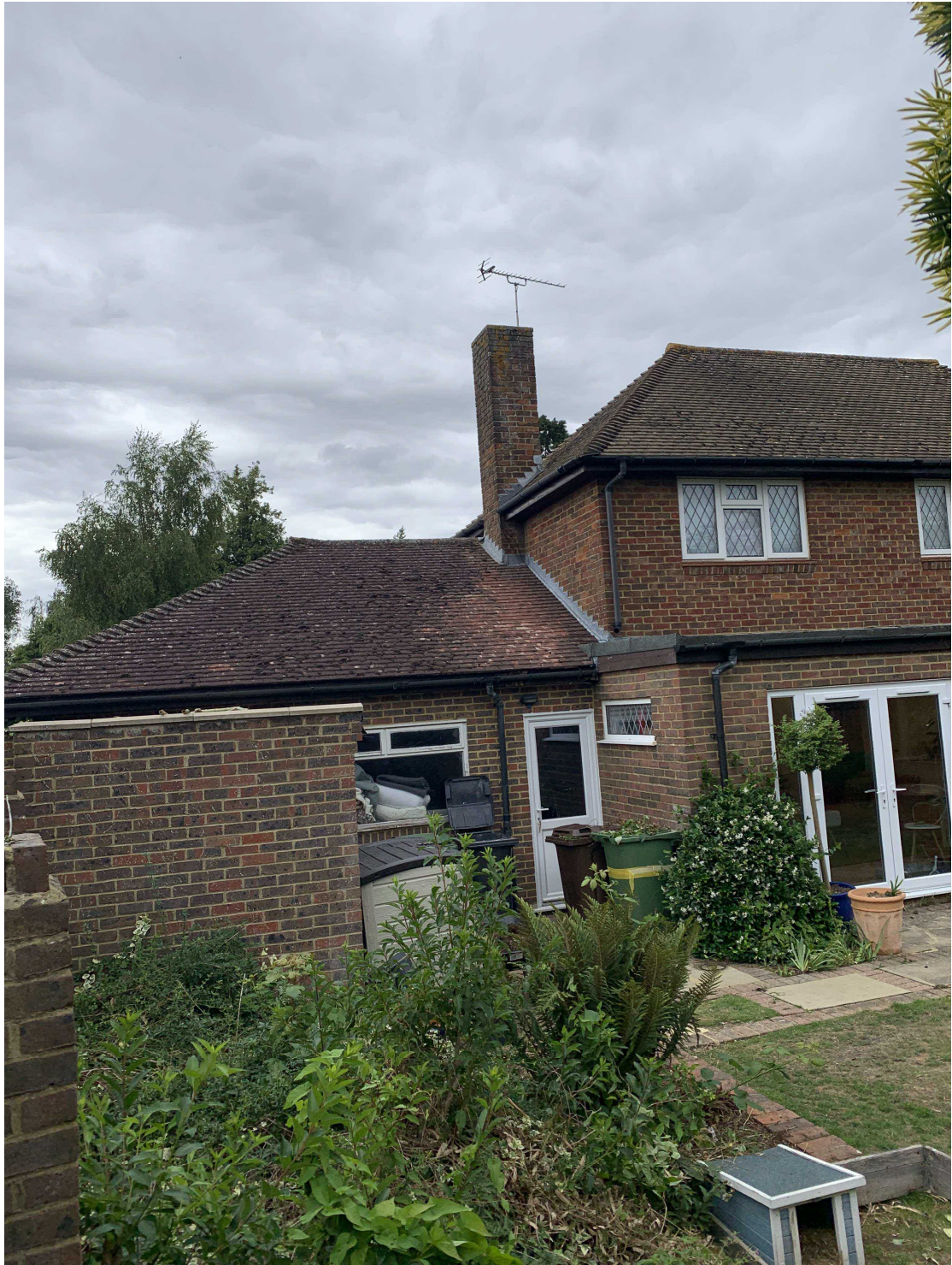
Rear Elevation as seen from directly behind the double garage
