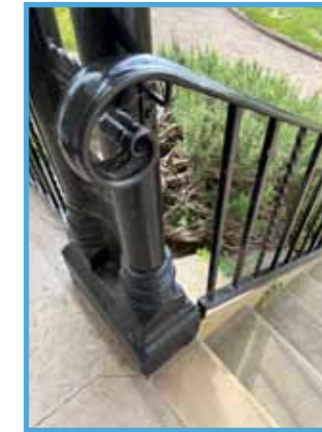
Existing handrail to entrance steps
