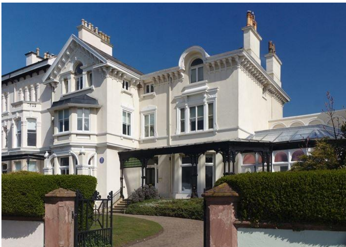
Figure 1 Photograph of No.13 Beach Lawn
