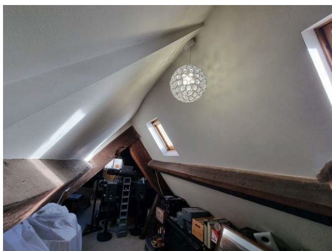
Fig 6: Purlins and roof structure on second floor .
