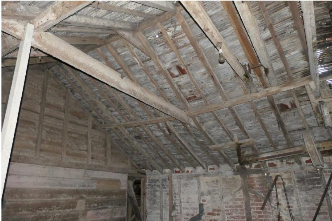
Photo 26 , internal view of building three's first level, looking west.
