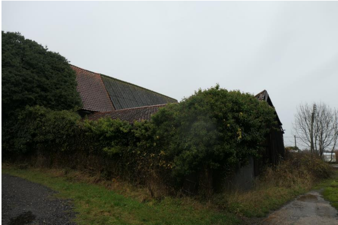
Photo 10 , north and east aspects of building one, looking northwest.
