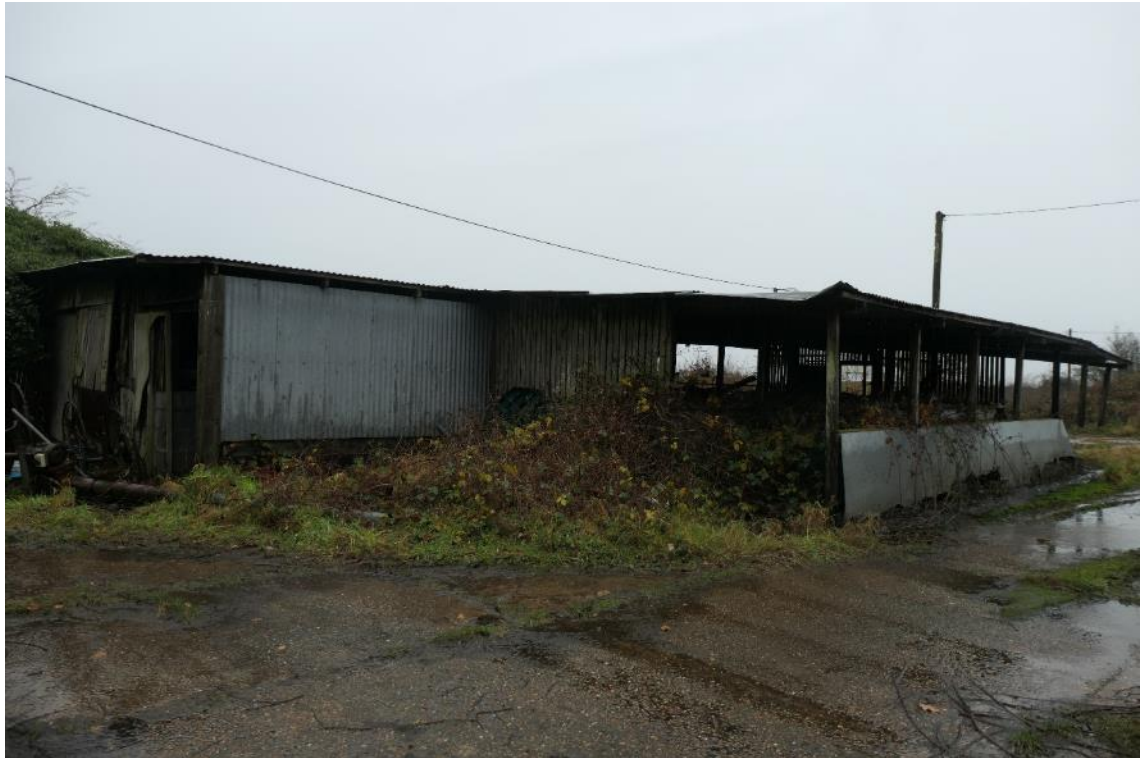
Photo 39 , west and south aspects of building eight, looking northeast.
