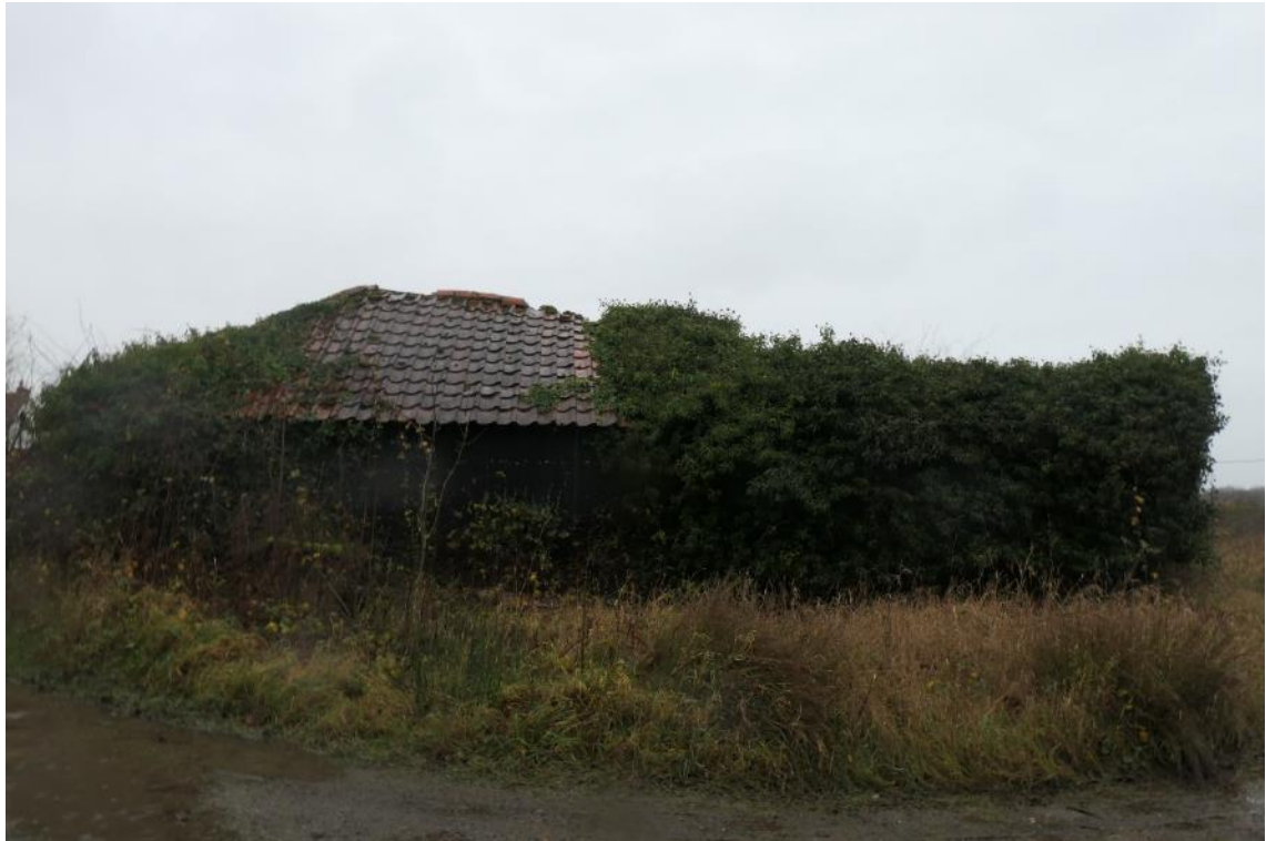
Photo 33 , eastern aspect of building five, looking east.
