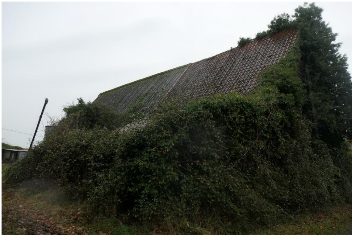
Photo 9 , west and south aspects of building one, looking northeast.
