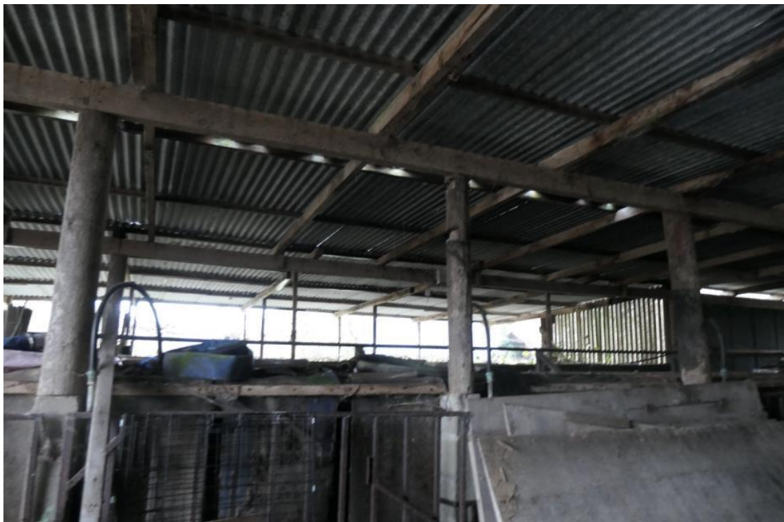
Photo 40 , internal view of building eight, looking south.
