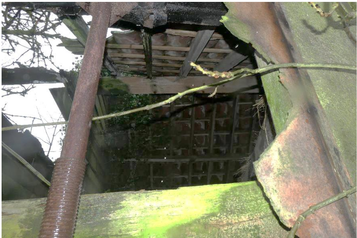
Photo 34 , internal view of building five, looking east.
