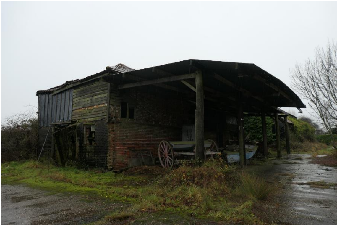
Photo 24 , north and west aspects of building three, looking southeast.
