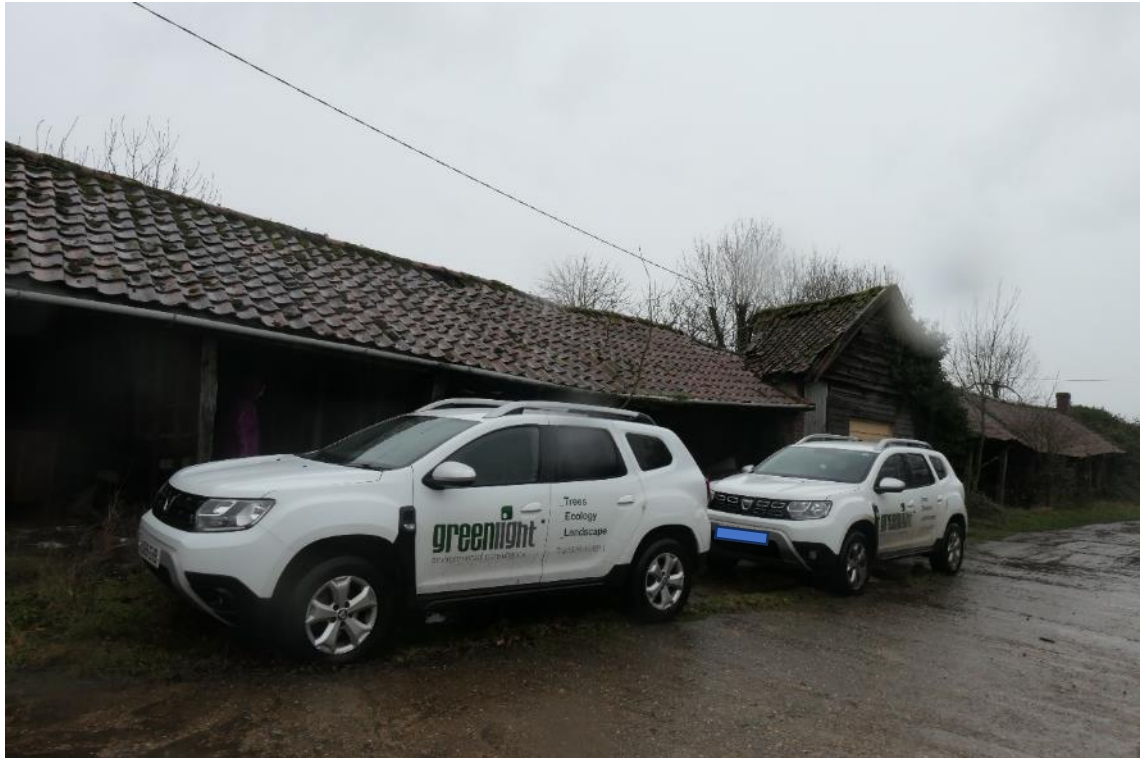
Photo 29 , western aspect of building one, looking southeast.
