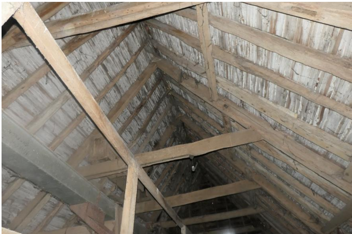
Photo 11 , internal view of building one, looking south.
