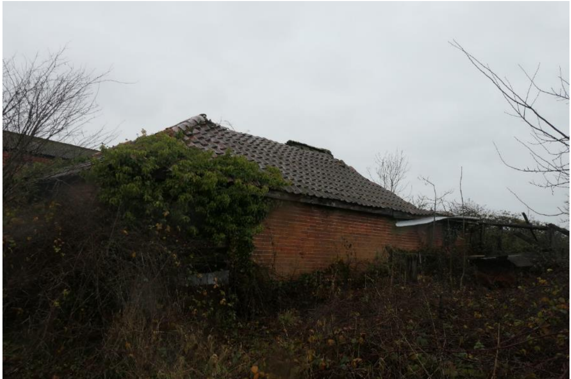
Photo 35 , south and east aspect of building six, looking northeast.
