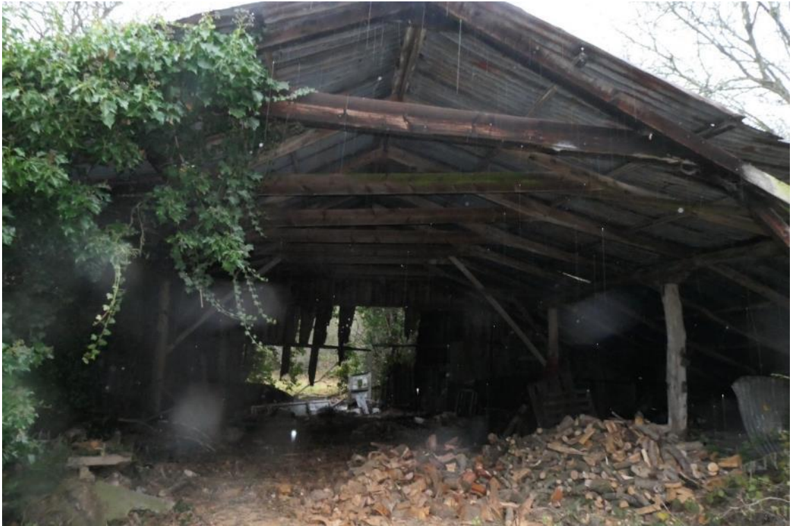
Photo 37 , east aspect of building seven, looking west.
