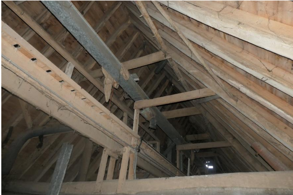
Photo 12 , internal view of building one, looking north.
