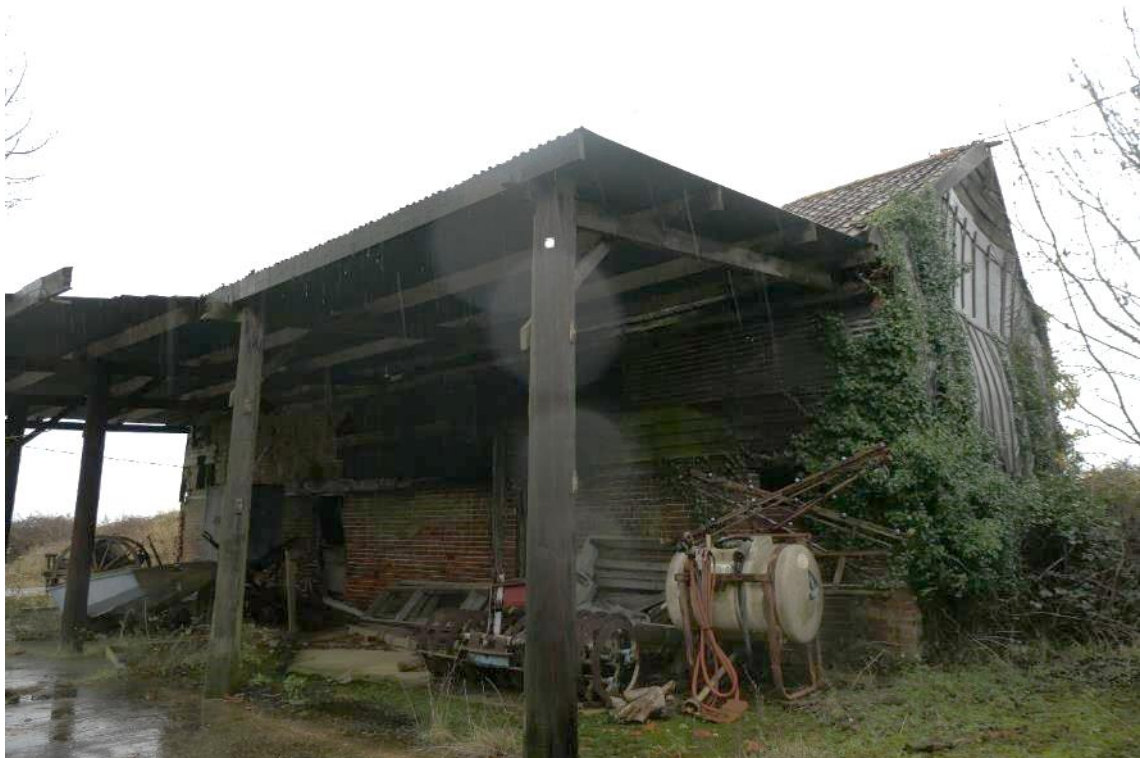
Photo 25 , south and west aspects of building three, looking north.
