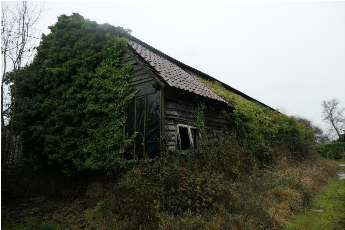
Photo 16 , north and west aspects of building two, looking southeast.
