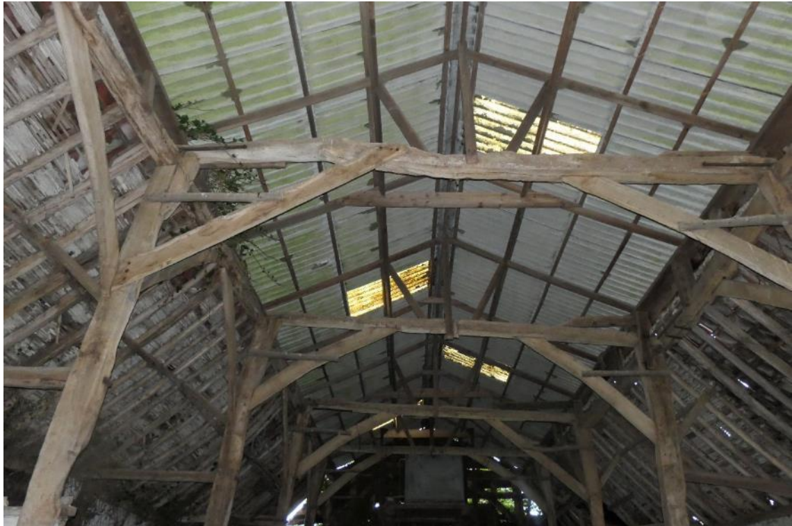
Photo 17 , internal view of building two, looking north.
