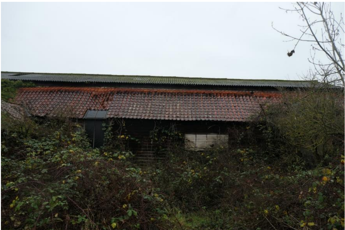
Photo 17 , eastern aspect of building two, looking west.
