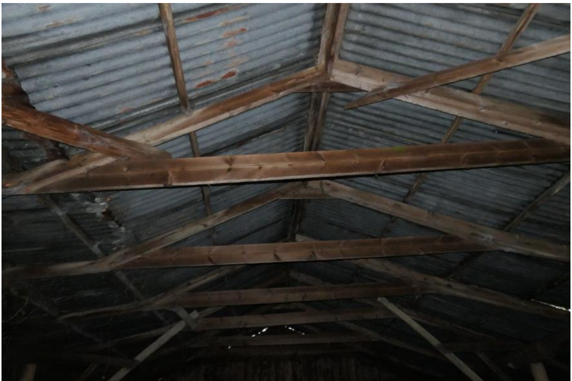
Photo 38 , internal view of building seven, looking west.
