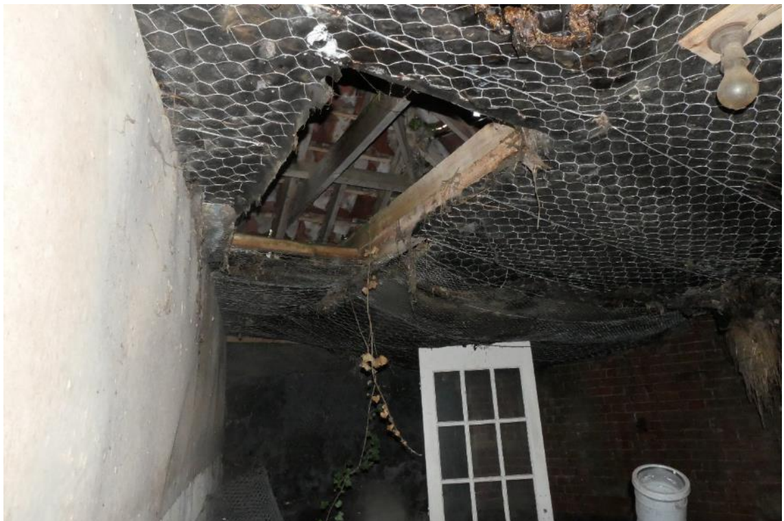
Photo 36 , internal view building six, looking southeast.
