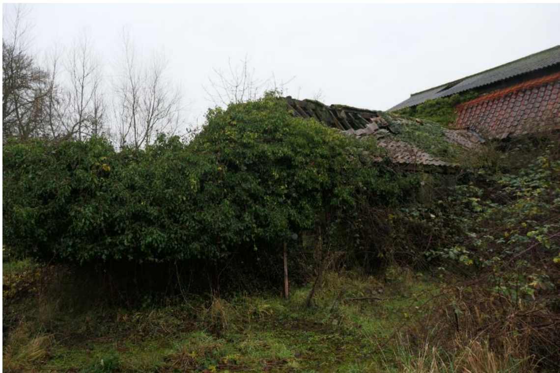
Photo 22 , north and east aspects of building two extension, looking southwest.
