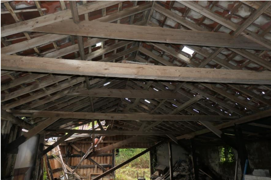
Photo 14 , internal view of building one extension, looking east.
