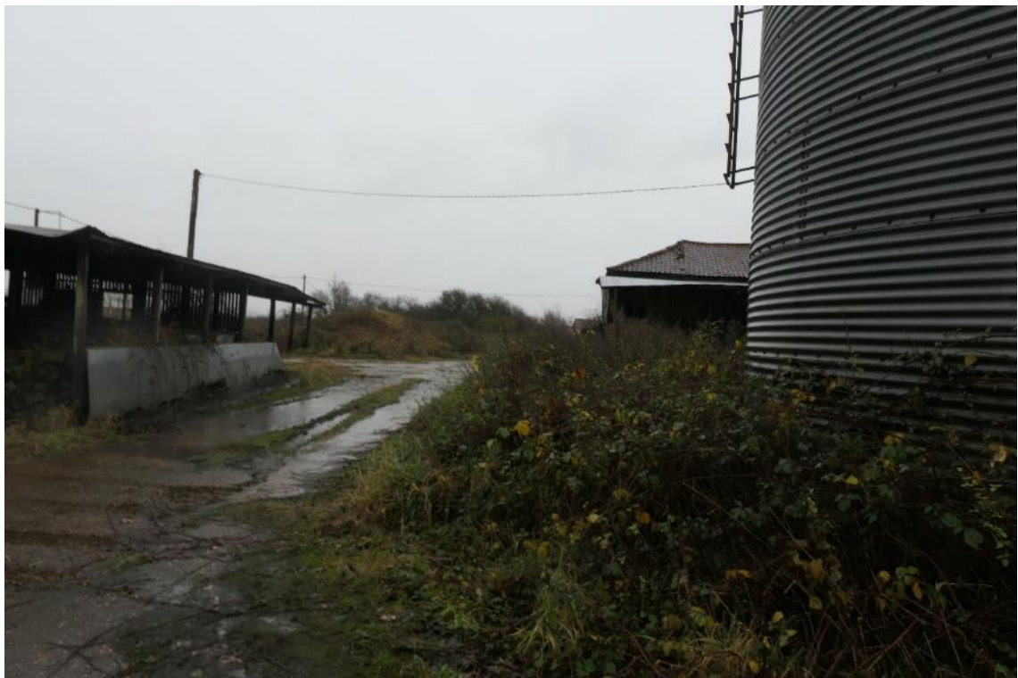
Photo 4 , hardstanding, building three, eight and nine, and bramble scrub, looking northeast.
