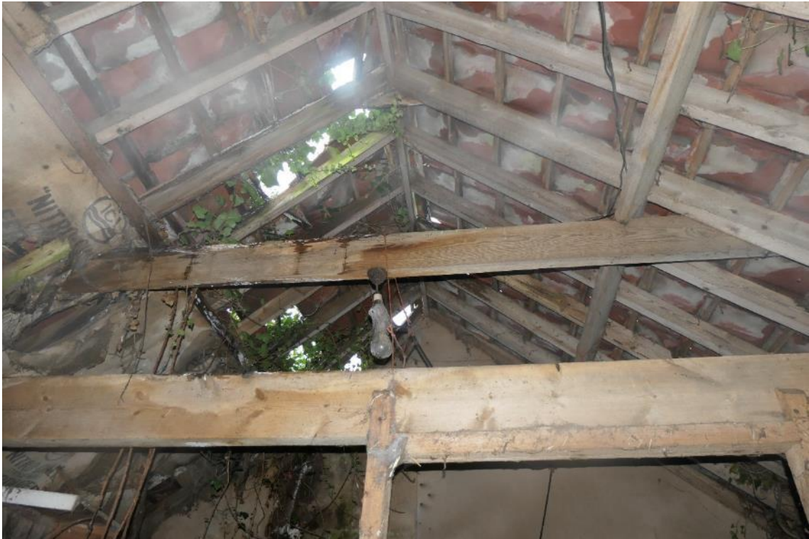
Photo 23 , internal view of building two extension, looking east.
