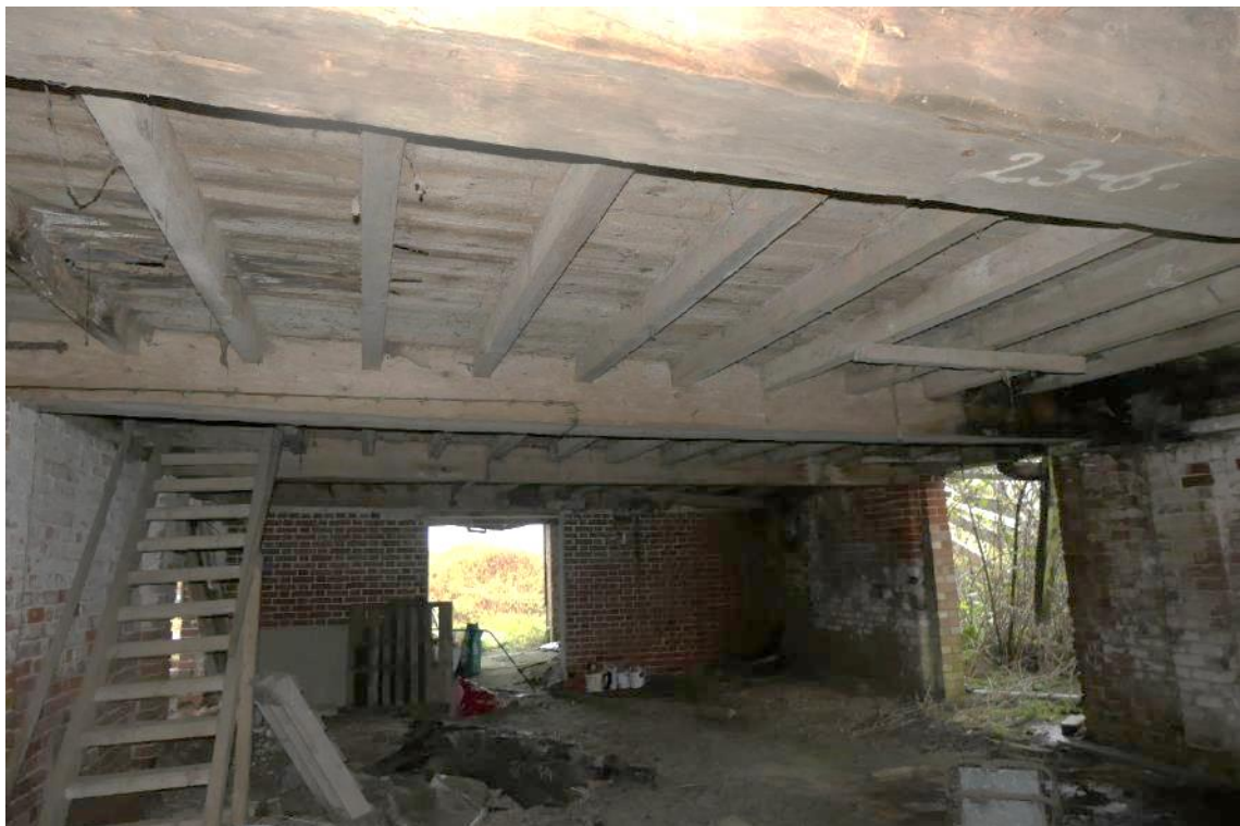
Photo 27 , internal view of building three's ground level, looking south.
