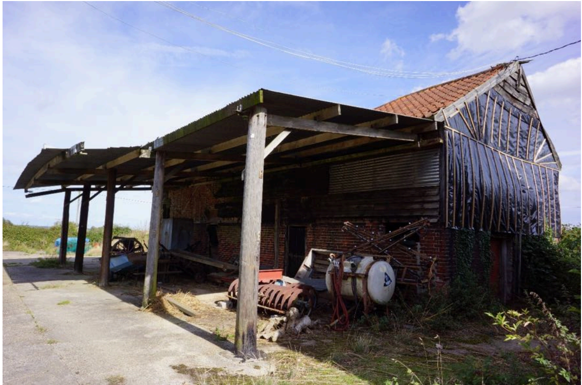
Photo 5 , view of the mill, looking northeast.
