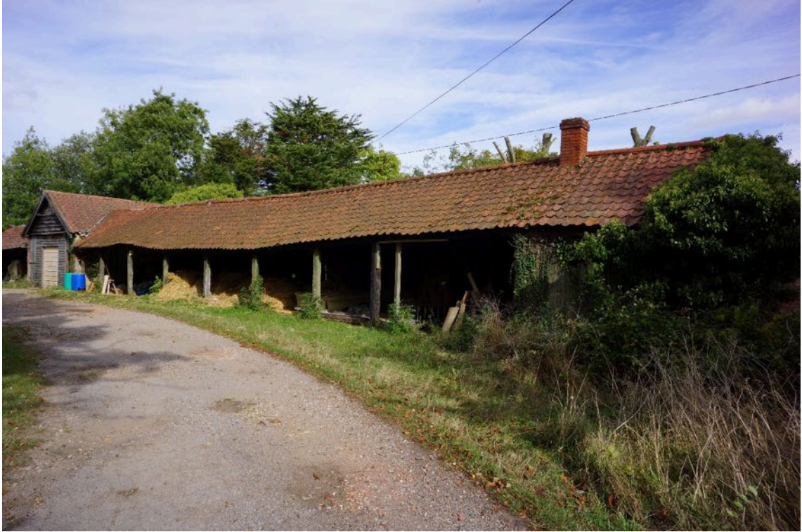
Photo 17 , view of the cart lodge, looking northeast.
