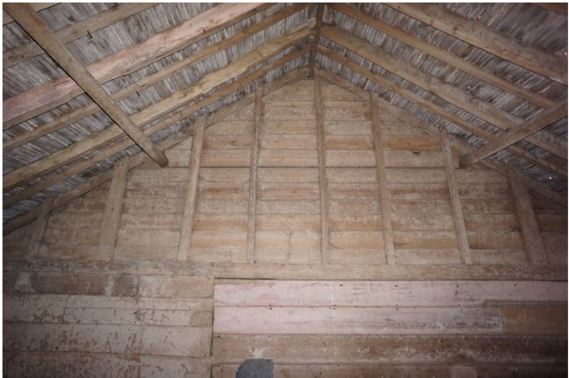
Photo 6 , internal view of the mill, looking south.
