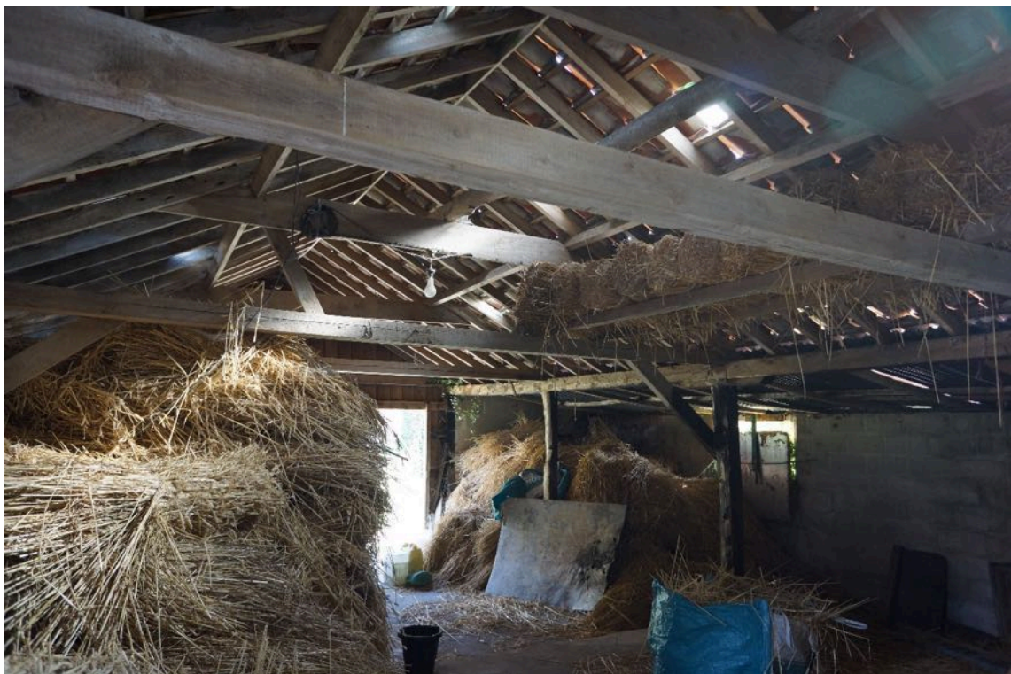
Photo 10 , internal view of the grain store eastern extension, looking east.
