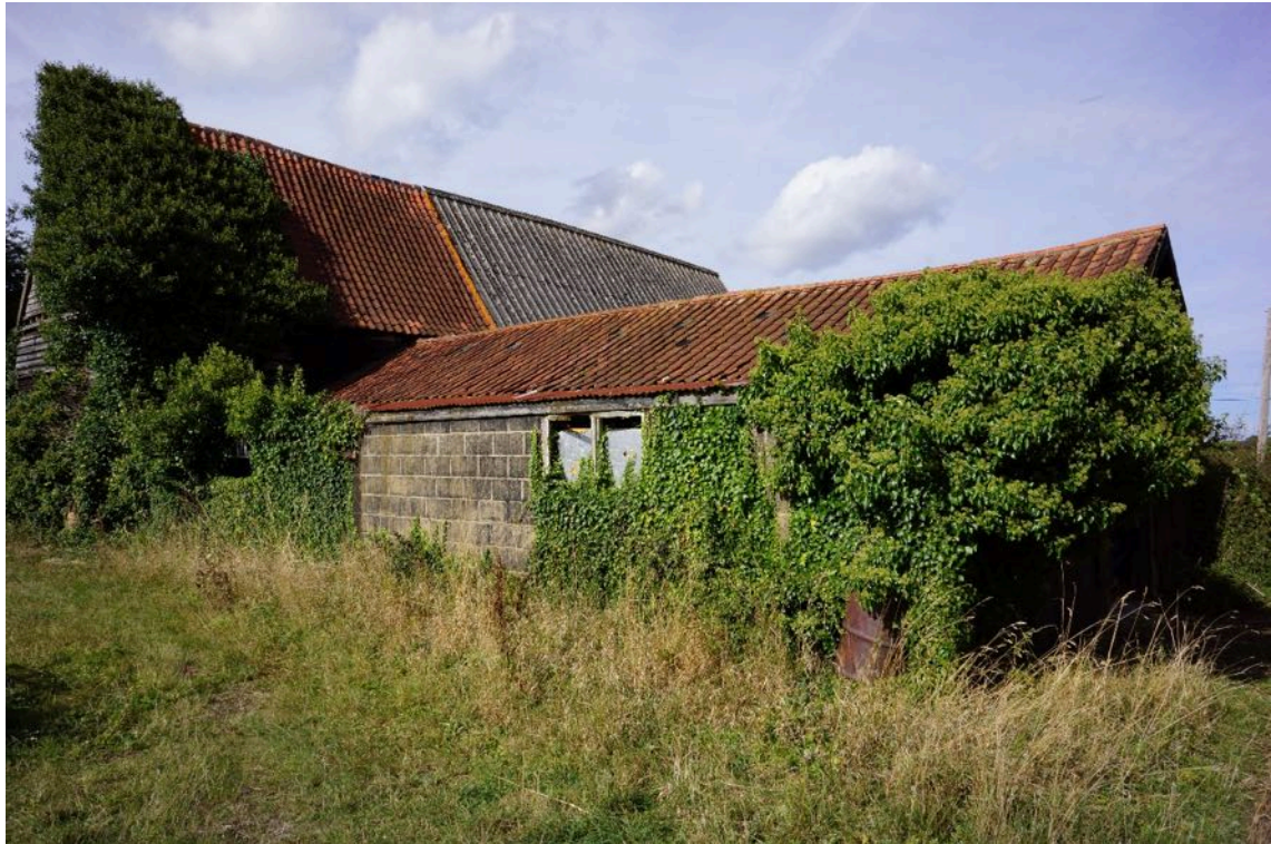
Photo 9 , view of the grain store and eastern extension, looking northwest.
