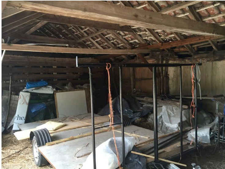
View internally of the northern unit.
