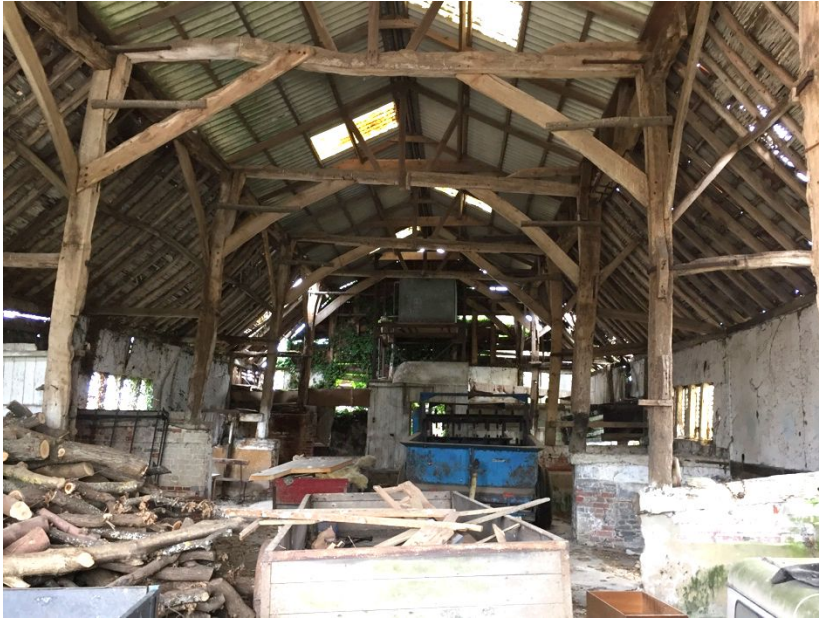
View internally from the south of the barn.
