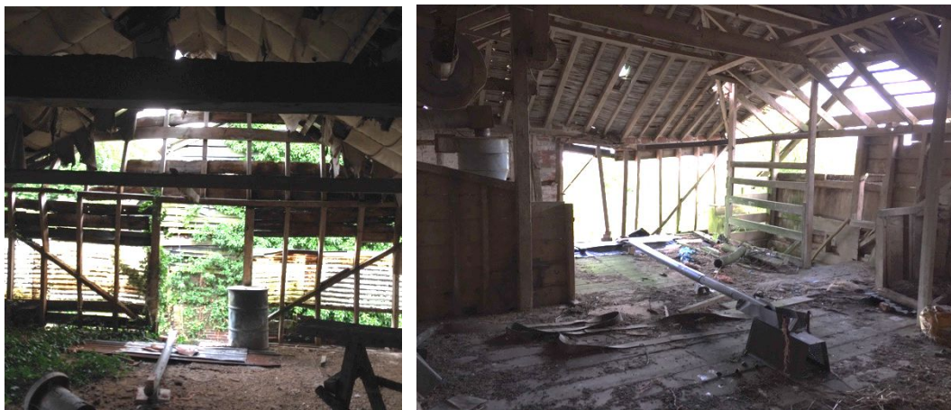
View of the exposed timber frame upstairs.
