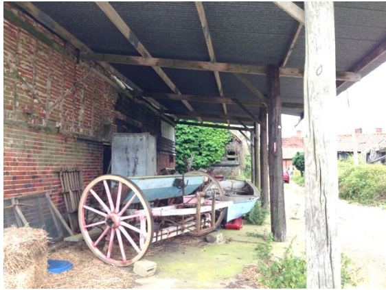
View of the covered overhang.
