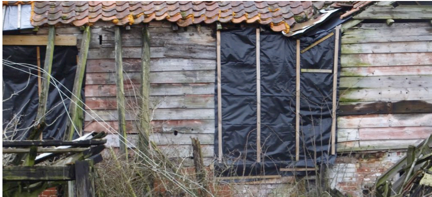
Section of easterly wall previously protected from the elements indicating traces of red ochre
