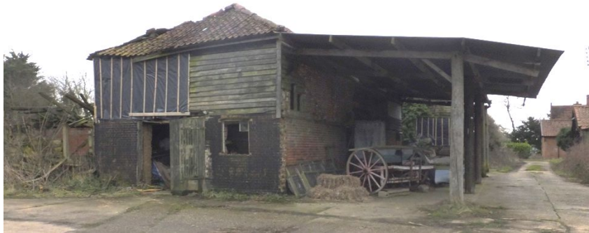
View from the north of the Mill.
