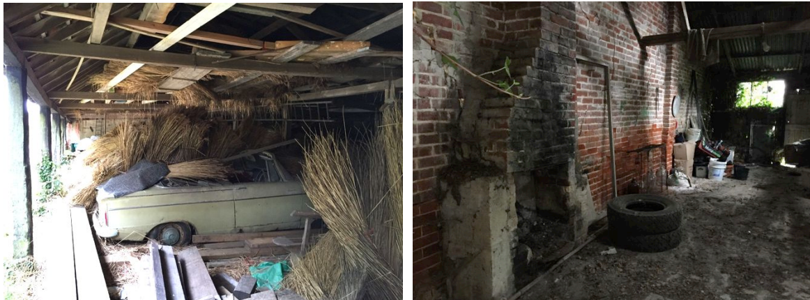
View internally of the southern unit and southerly brick section.
