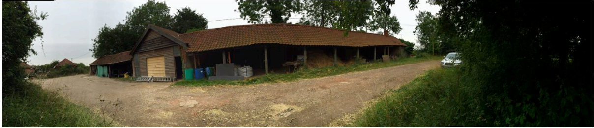
Front elevation of the cartlodge and the existing accessway.
