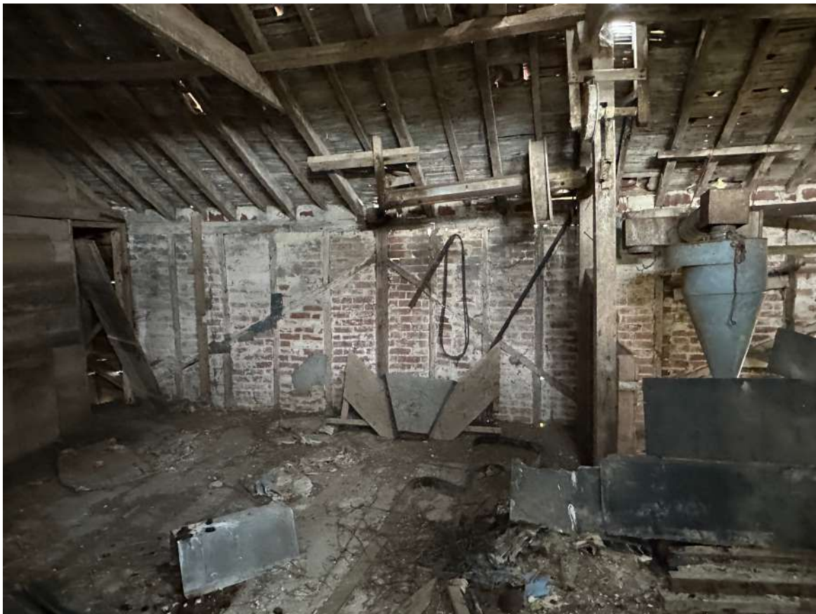
The 'Old Mill' Building with Brick Ground floor walls (Above) and timber frame with Brick infill to the first floor (below)
