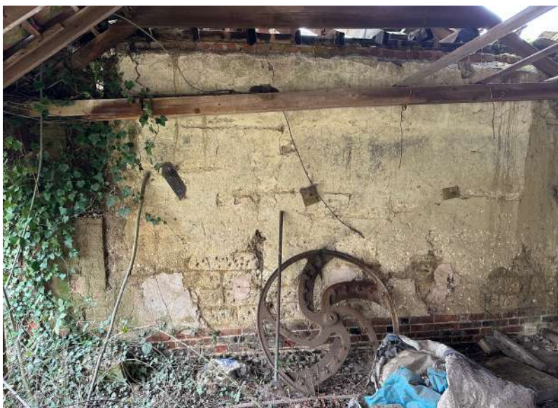
Cartlodge - Showing the garage section roof now partially collapsed (above) and Clay lump wall still intact (Below)
