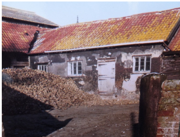
Forming northern side to courtyard, part masonry, part timber framed, only part of south and north walls now standing.
