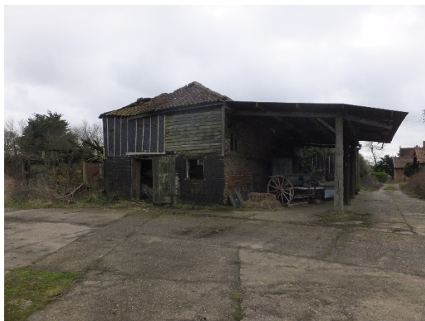
Forming northern side to courtyard, part masonry, part timber framed, only part of south and north walls now standing.
