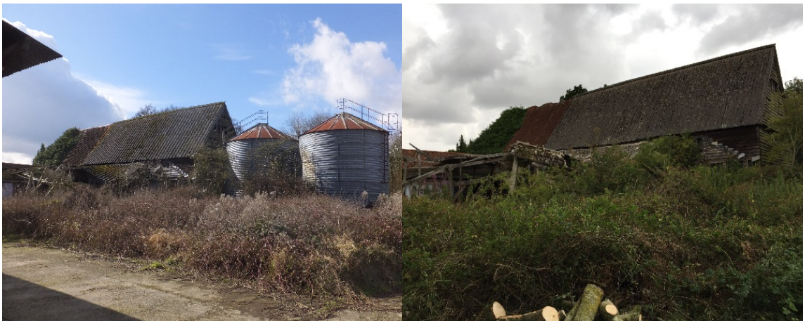
Presenting as a ten bay building, but actually two barns constructed end to end, main axis north/south, now containing corn storage and drying equipment, with a lean-to structure at southern end, west side. Major extensions in timber framed construction to east side now derelict.
