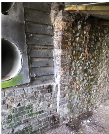
(Straight joint in plinth, west side)
