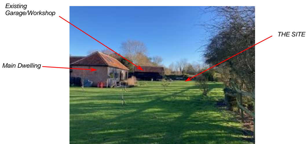
Figure 2 – View of existing dwelling from Garden
