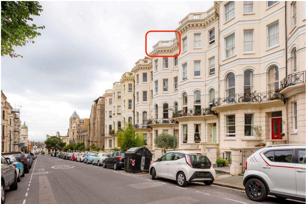
Image 1 (view from north)
