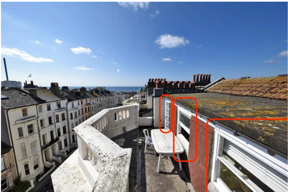
Image 4 (view from roof terrace, highlighting windows and doors that need replacing)
