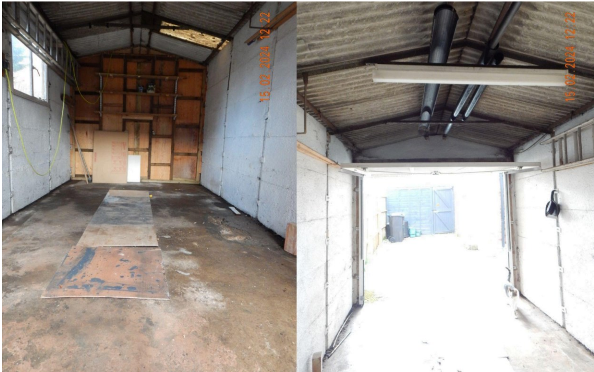
Image 7 – Internal view from within the internal areas of the detached garage
