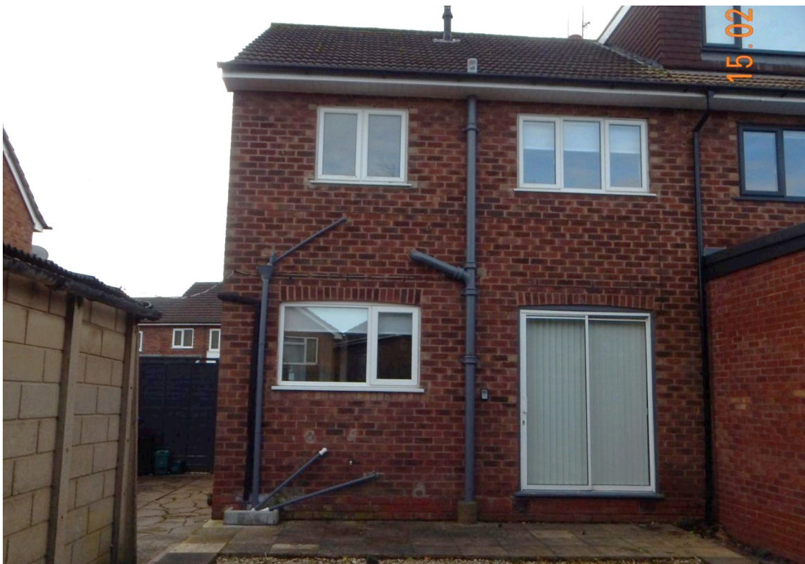
Image 2 – Rear North facing elevation of the main dwelling
