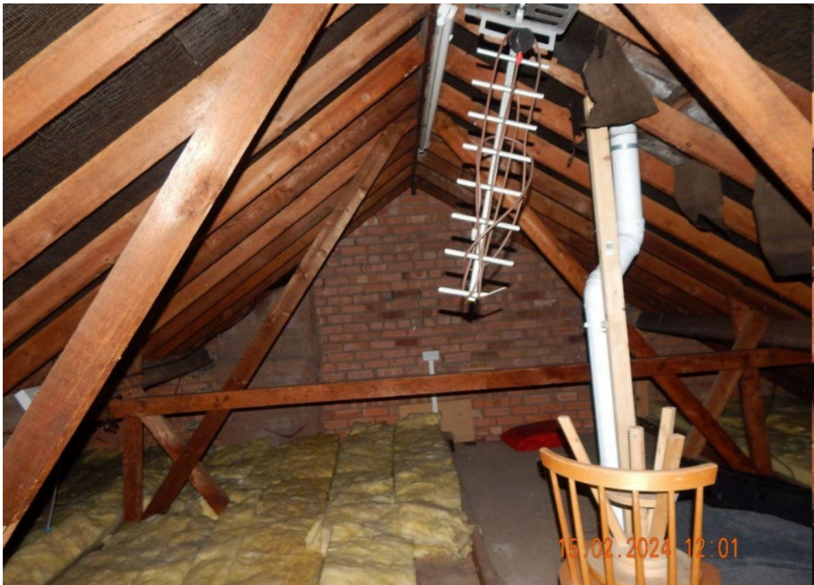
Image 5 – Internal view from within the roof void spaces of the property
