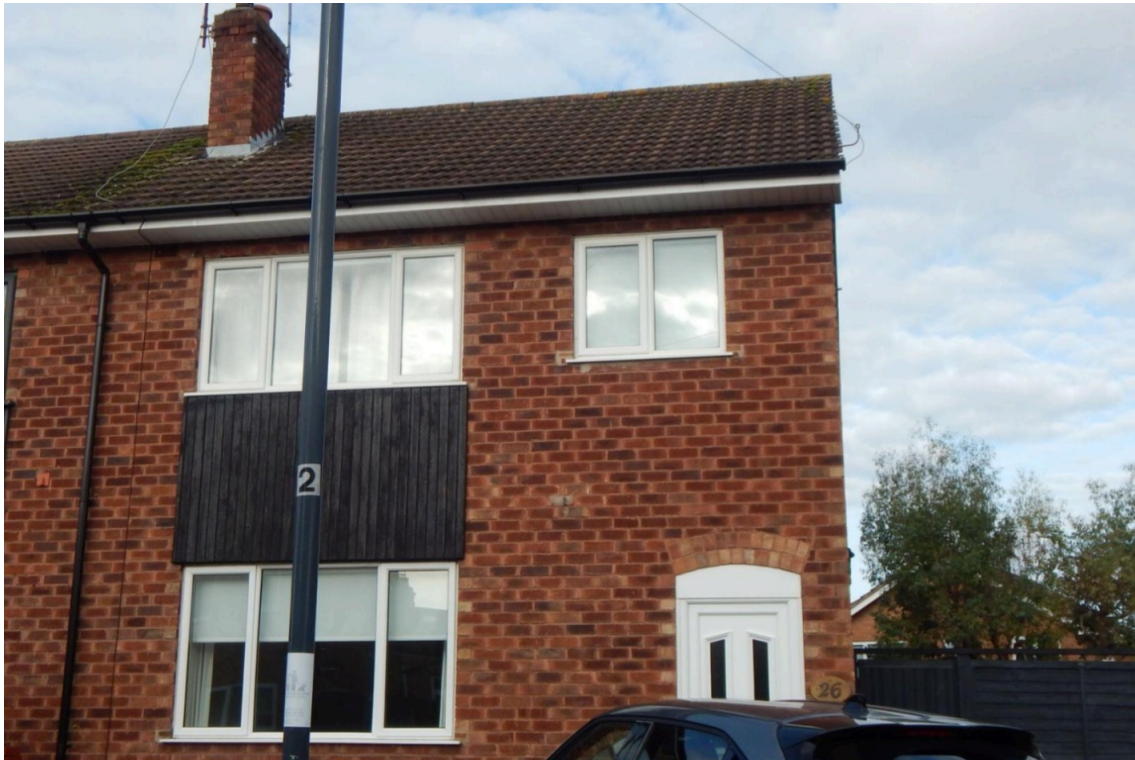
Image 1 – South facing elevation of the main dwelling
