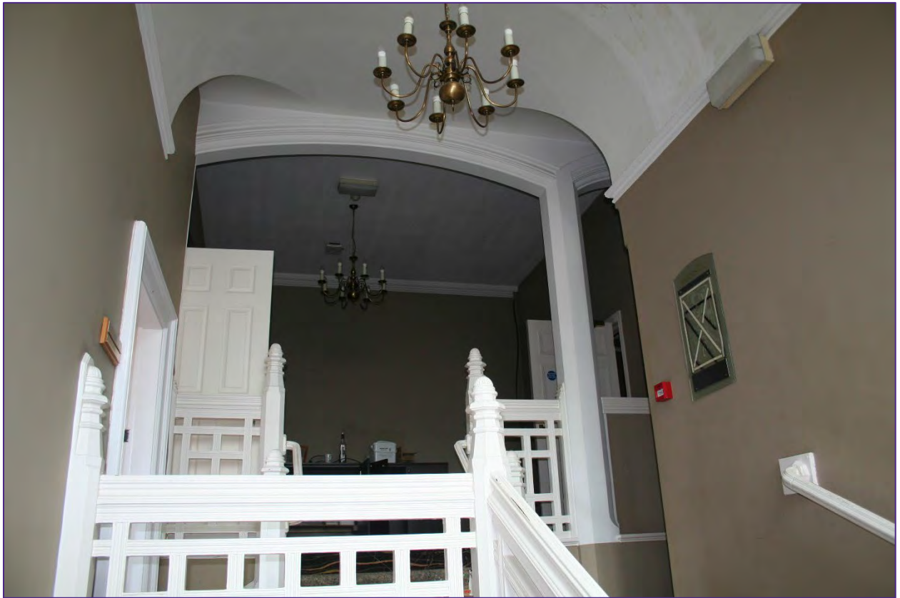
Plate 21: View from half landing on stairs towards arched landing.
