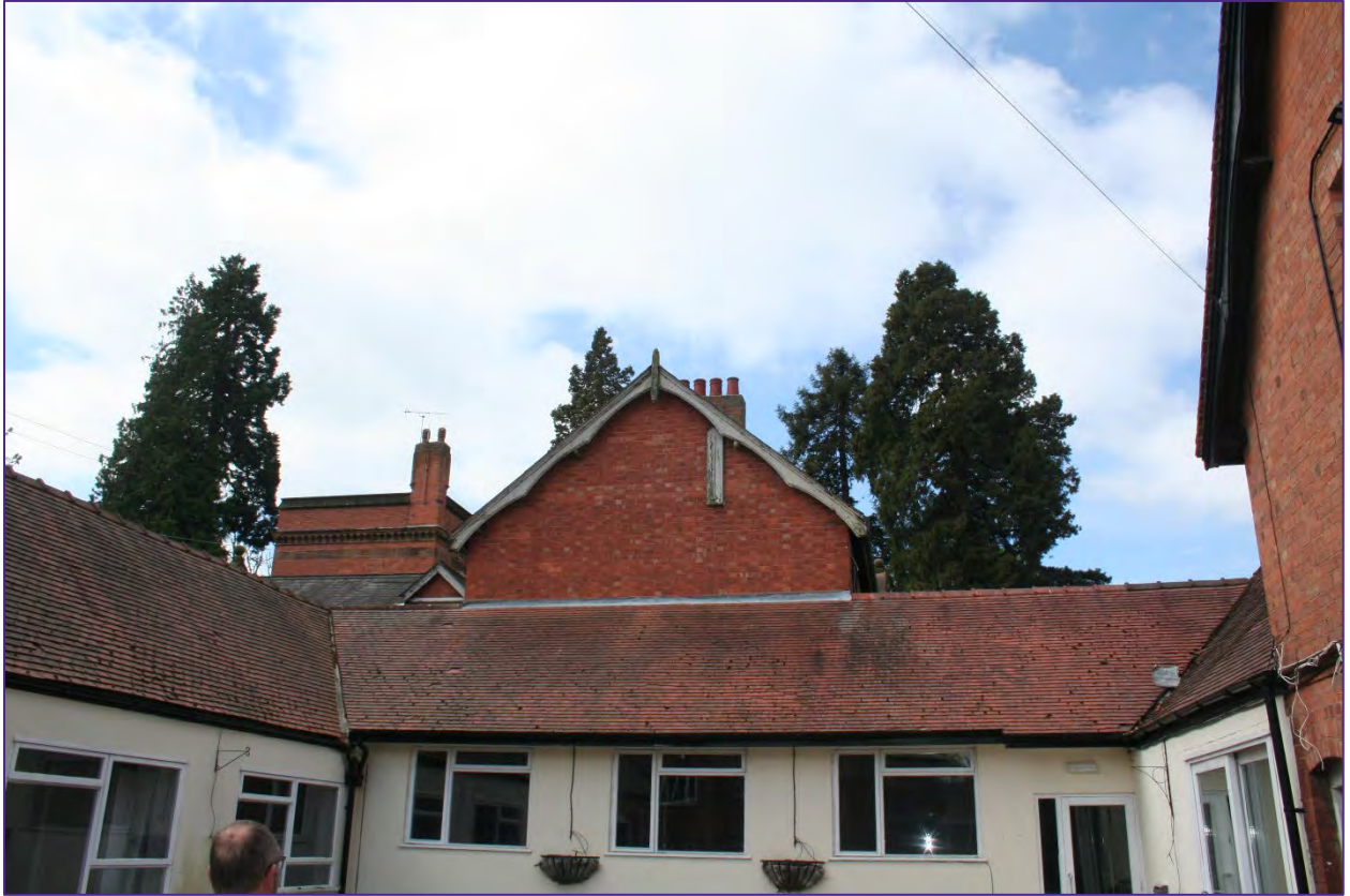
Plate 6: Gable end of the servants' wing with twentieth century extension below.
