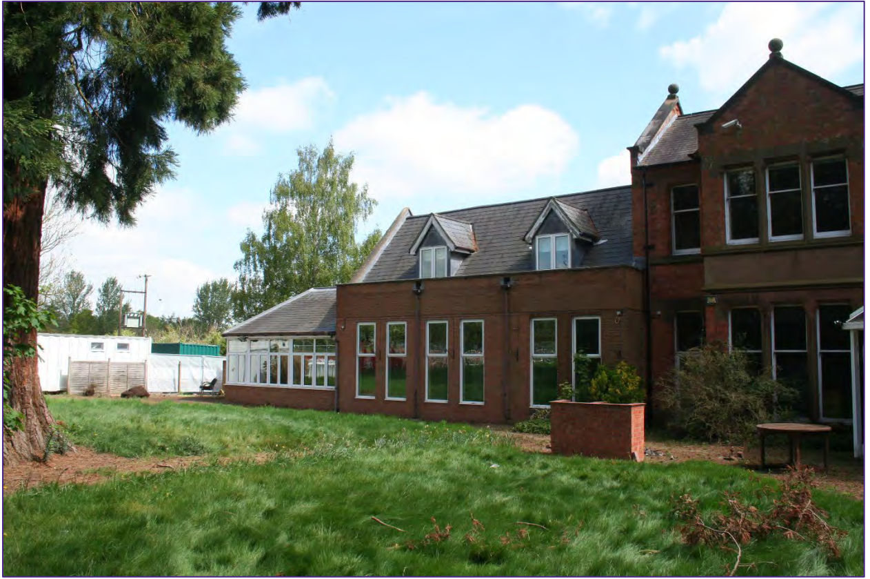
Plate 9: Post-war extensions to north-western corner of Woodside.
