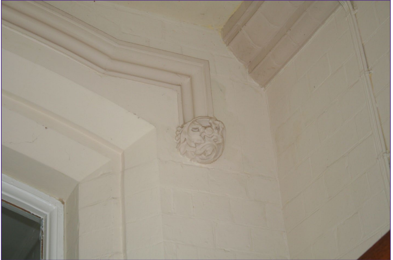
Plate 13: Hoodmould with headstops on original nineteenth century entrance into Woodside.
