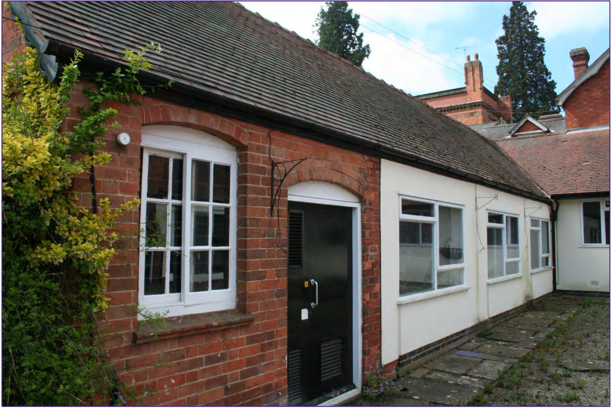
Plate 5: Former carriage building now converted to offices.
