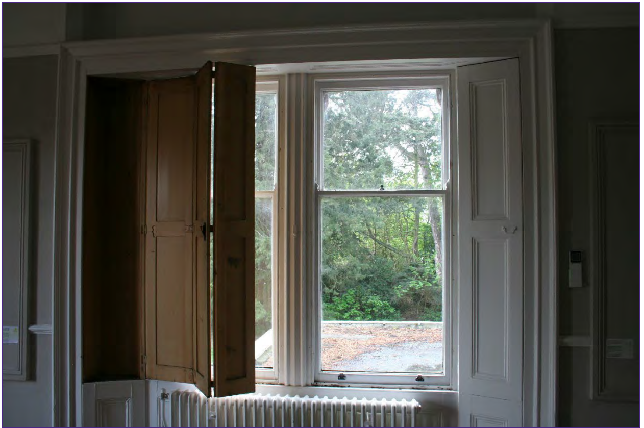
Plate 26: Timber panelling, shutter boxing and shutters in bedroom.
