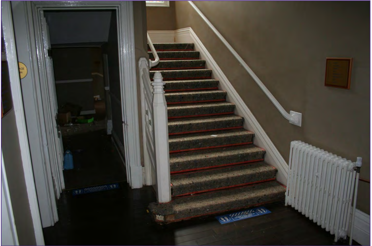
Plate 19: Base of the principal stairs with under stairs corridor to the smoking room.
