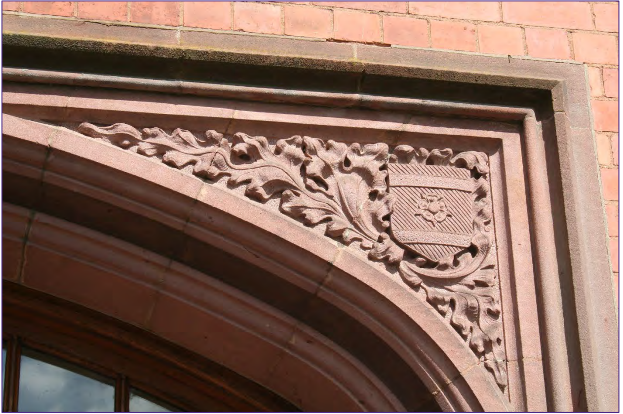
Plate 11: Three-centred sandstone doorcase with labelled drip mould, coats of arms and floriolate designs.
