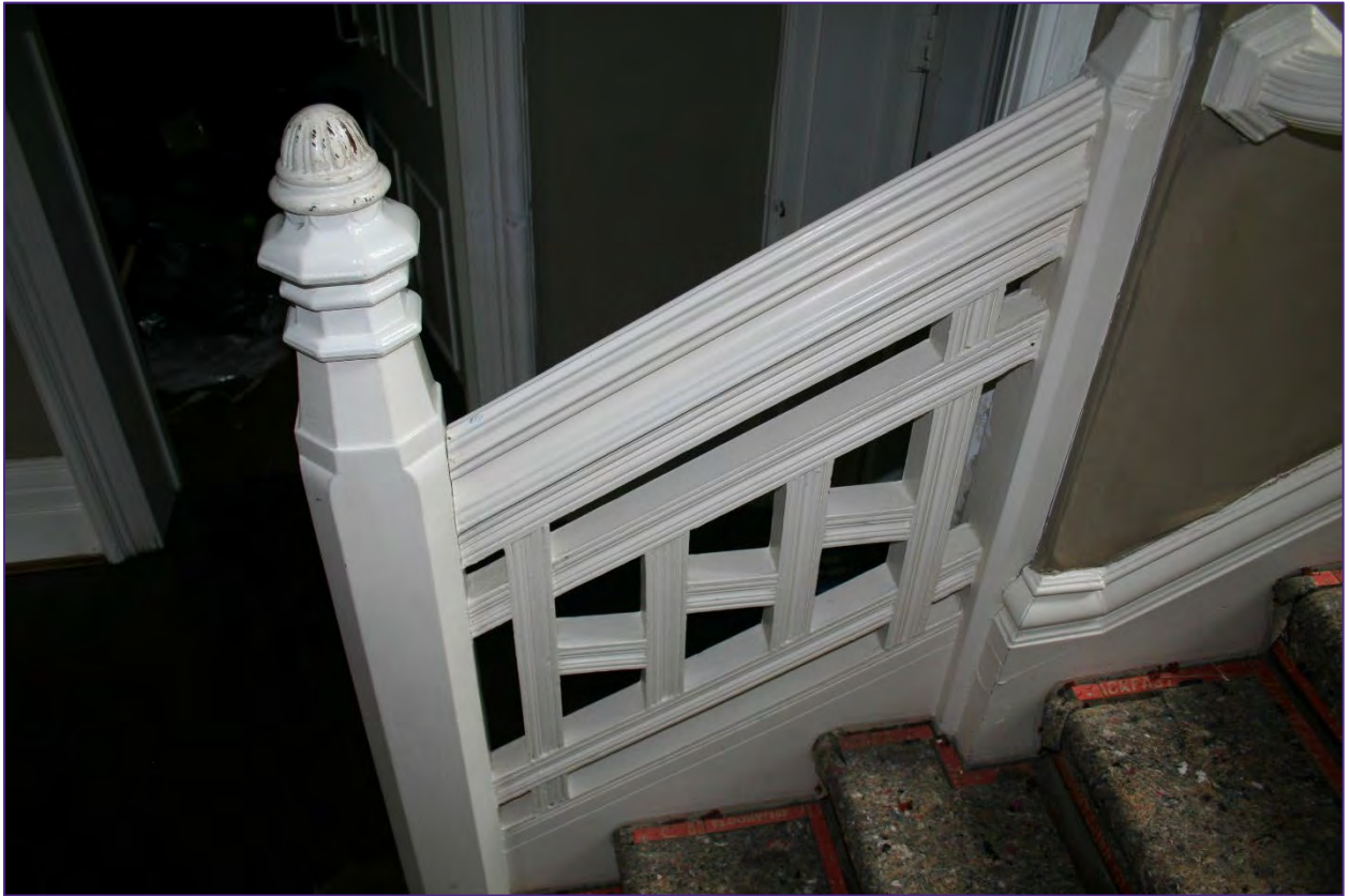
Plate 20: Timberwork on staircase.
