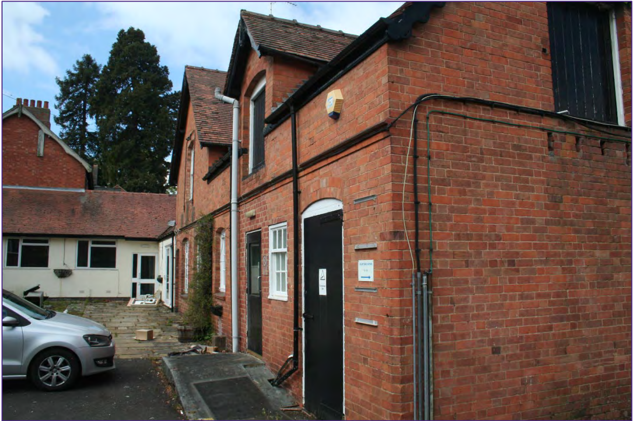
Plate 4: The former stables and farm buildings. Later link to former carriage building centre left.
