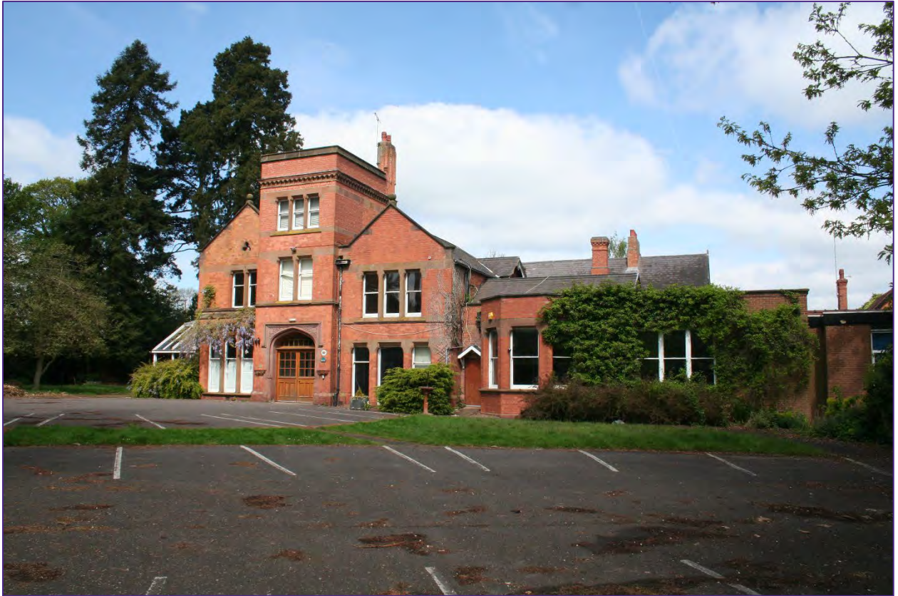
Plate 1: Woodside viewed from the south within car parking area.
