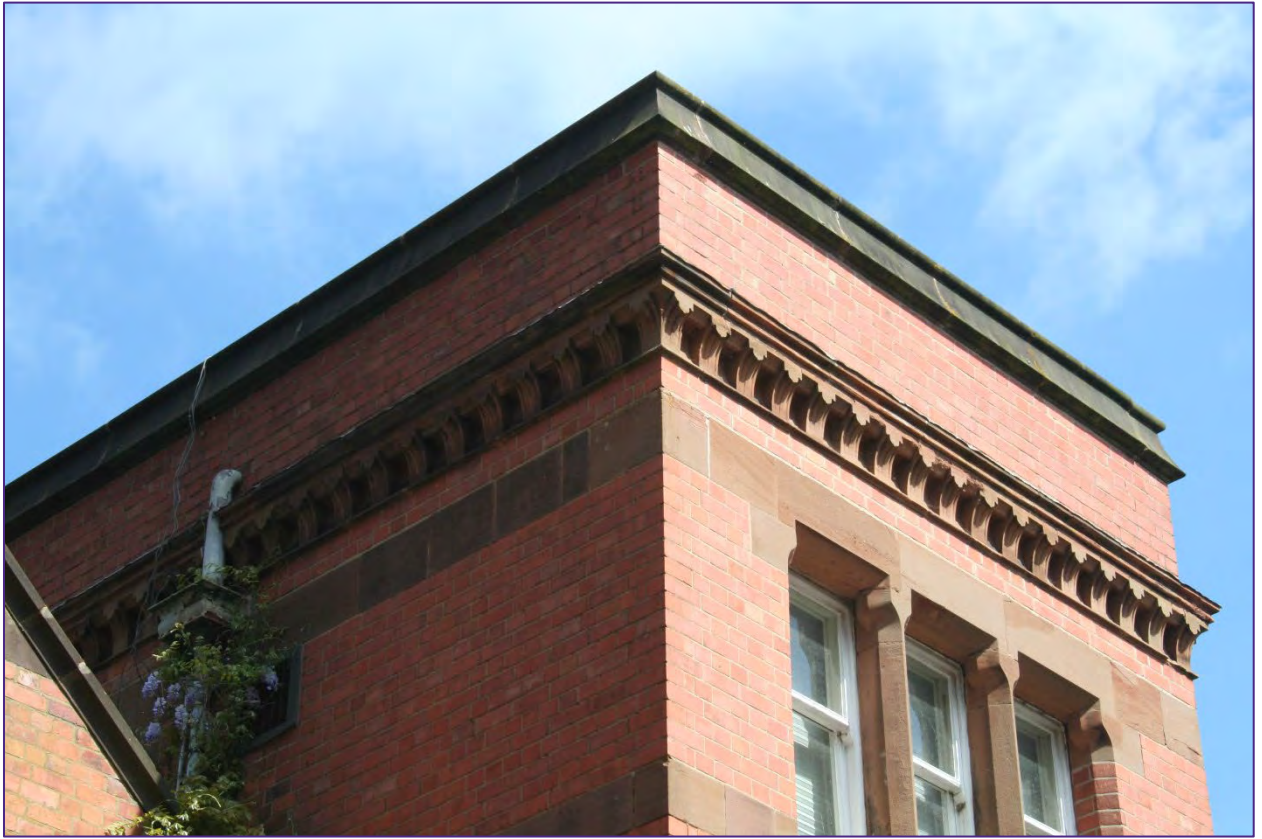
Plate 12: Second floor of entrance tower with sandstone detailing and parapet.
