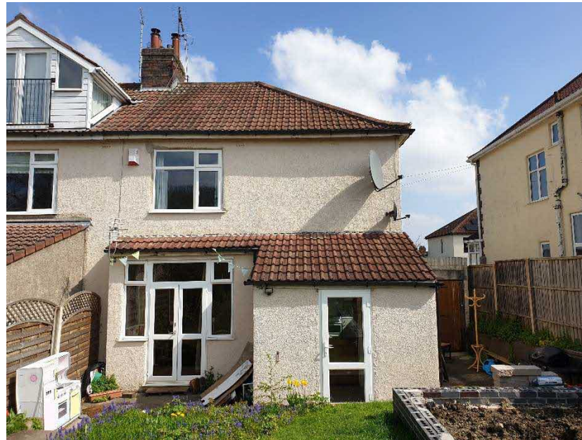
Site photographs :: 47 Laurie Crescent, Bristol. BS9 4SZ
