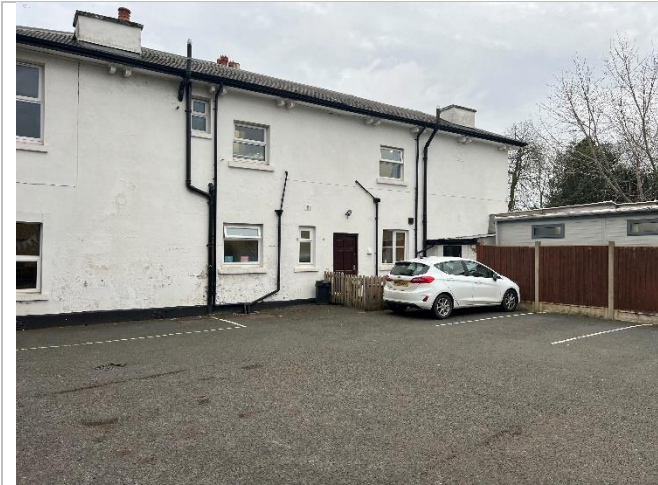
East elevation & car park
