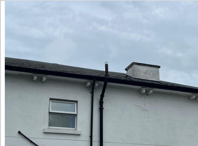
Slate roof and chimney
