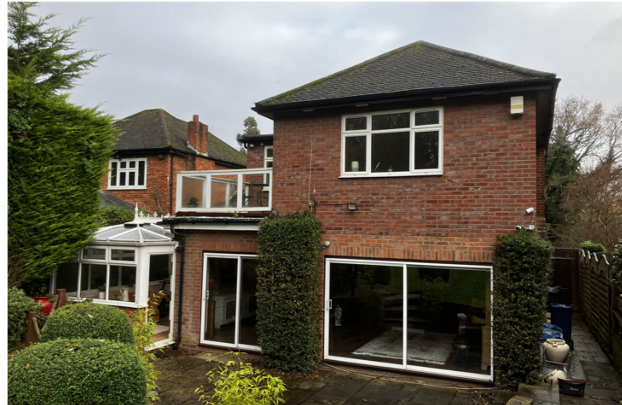
View of the rear elevation.
