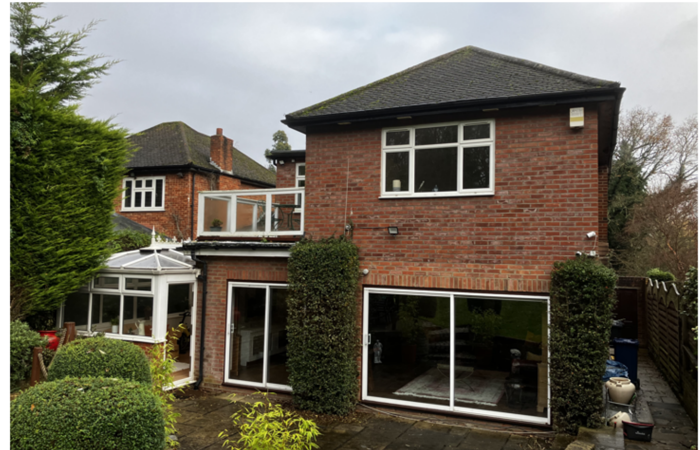
View of the rear elevation.
