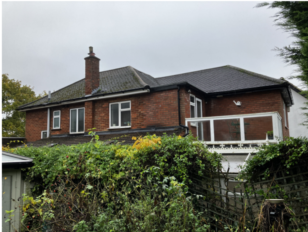
View towards the side elevation with balcony and conservatory.
