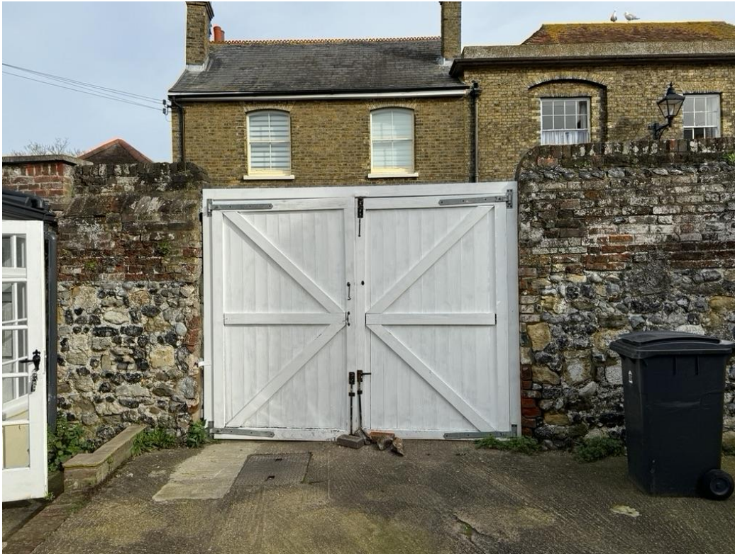
Photo (vii) – view of gates from inside garden courtyard
