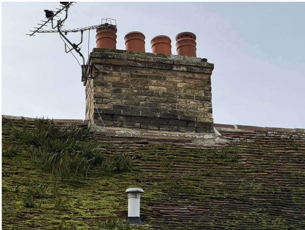
Photo (v) – chimney stack
