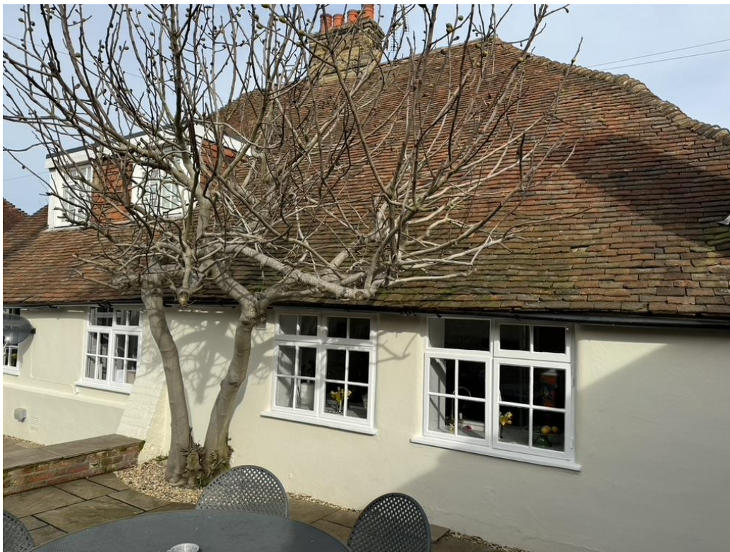
Photo (iii) – rear elevation (no works proposed)
