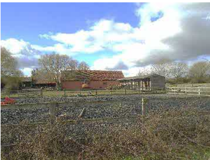
Figure 1 The stables looking from a distance to the west (left) and south (right)
