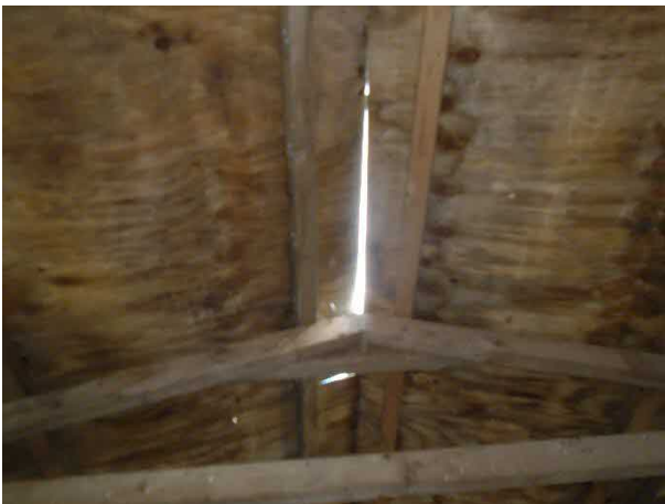
Figure 10. Interior of stable section. Top: gaps to internal ridge timbers (left) fly through areas above board divides (right). Bottom: Interior of stable used as log store (left), boarding and machine sawn timbers of empty stable (right).
