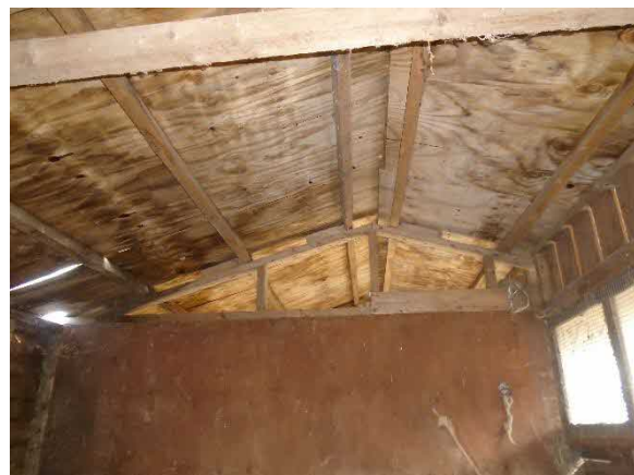
Figure 10. Interior of stable section. Top: gaps to internal ridge timbers (left) fly through areas above board divides (right). Bottom: Interior of stable used as log store (left), boarding and machine sawn timbers of empty stable (right).
