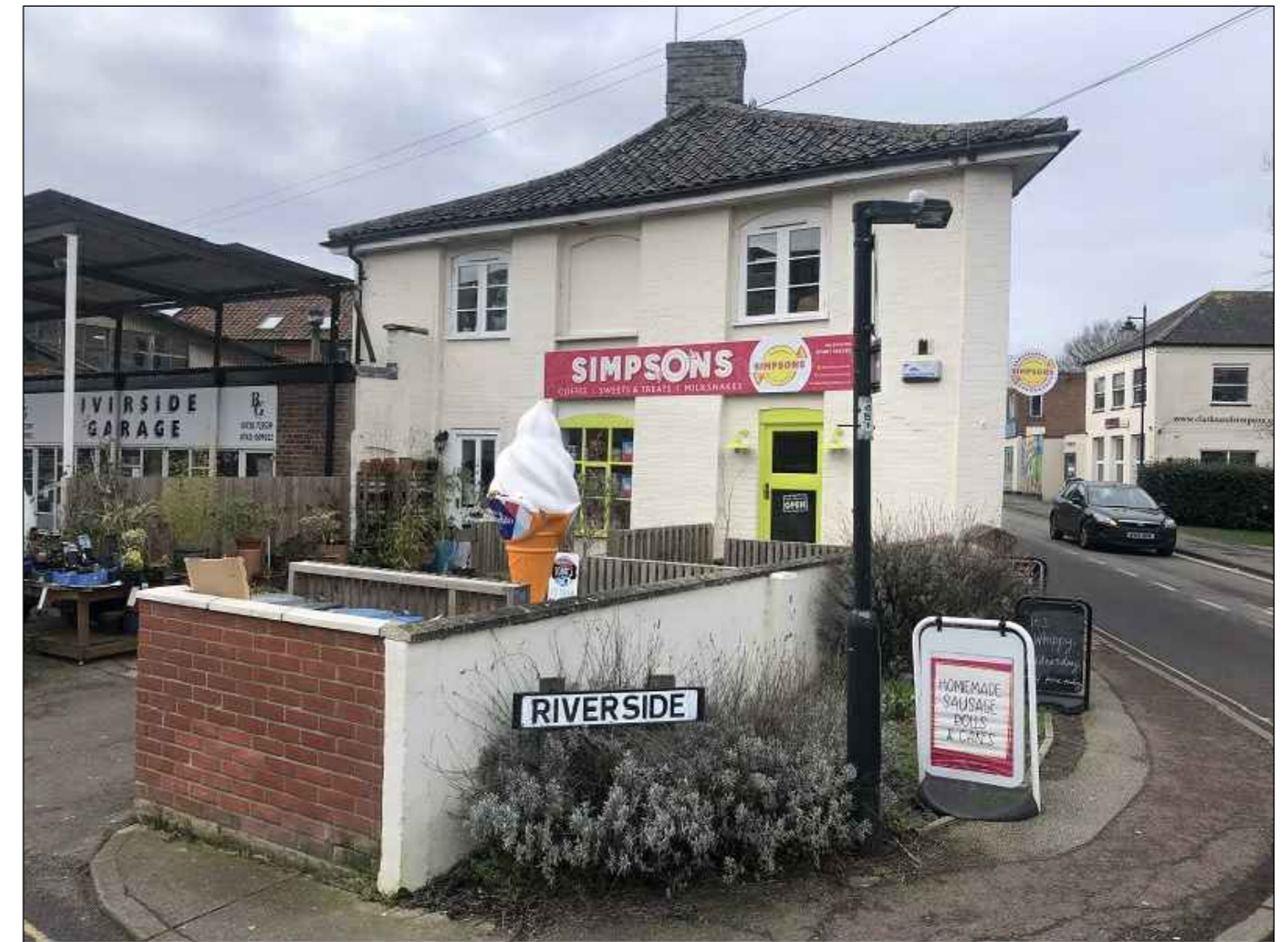
PHOTO FROM THE CORNER OF BRIDGE STREET AND RIVERSIDE
