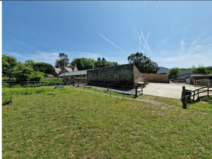
View of the cattery building (looking north) viewed from the field
