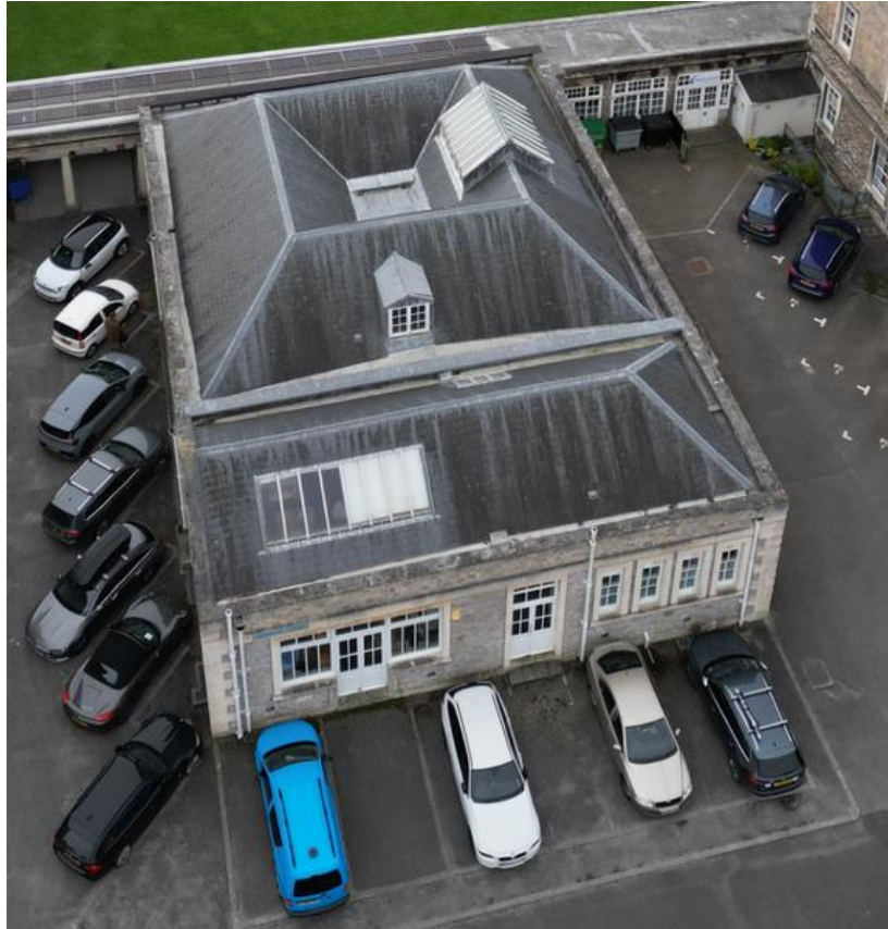
Figure 2. The building surveyed at this site.
