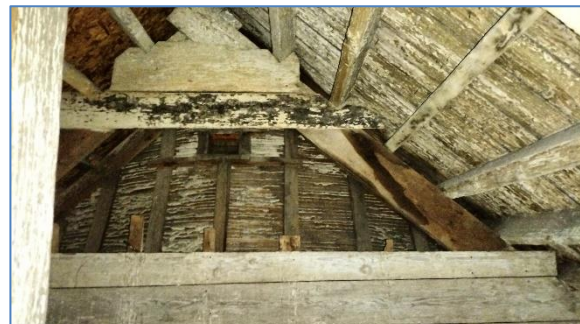
An example of the original timber frames.
