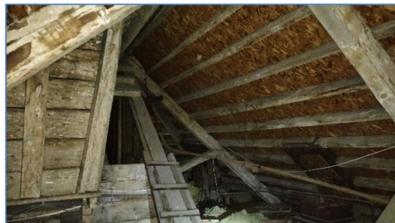
An example of the roof interior.
