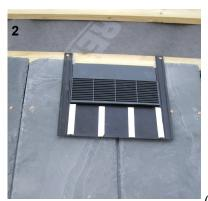
Insert the ventilator into the roof void and secure with slating nails into the batten (fig 2), ensuring that the vent sits closely onto the slates below. The Vent is designed for use with 25mm slating battens. Where a thicker batten is used then the back of the batten will need to be reduced to 25mm where it passes across the installed vent. Where the thickness of the slates on either side of the vent is greater than 8mm, then the same trimming of the batten may be necessary.
