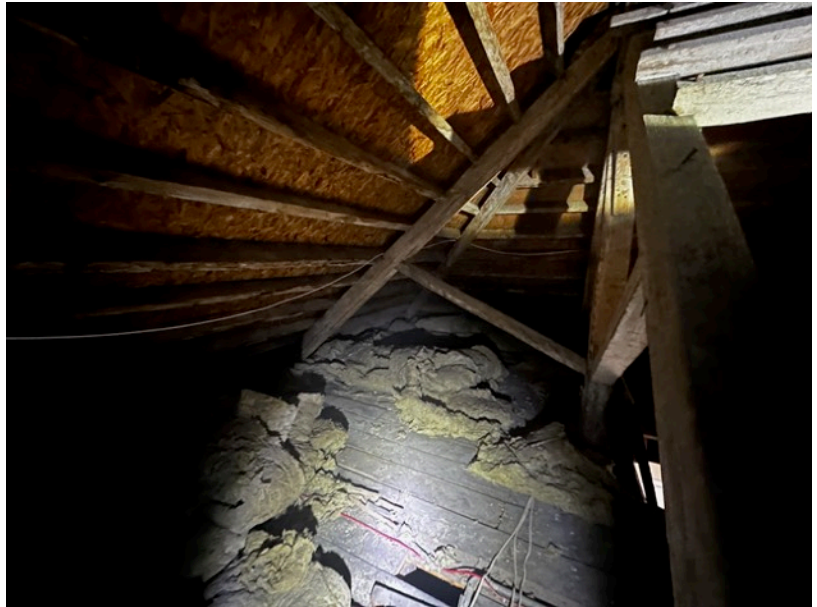
Roof space - note the OSB board sarking
