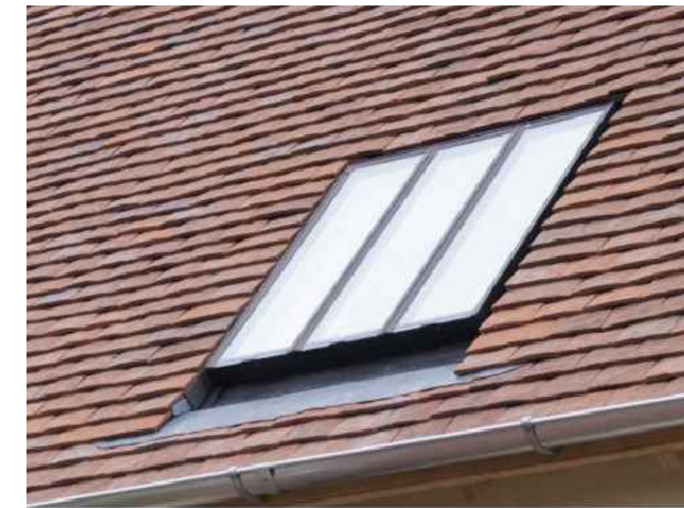
IMAGE REFERENCE - DOUBLE GLAZED 'CONSERVATION' ROOF LIGHTS
