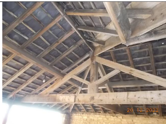
Plate 11: Building B, showing the internal timber framework.
