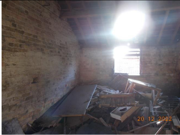
Plate 3: Building A, showing one of the glassless windows in a stall.
