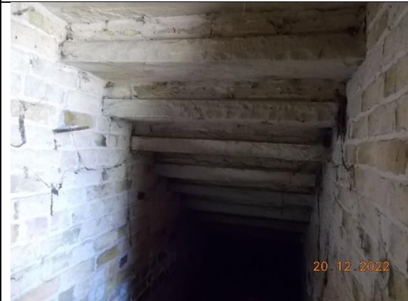
Plate 13: Building C, showing the space beneath the stairs.
