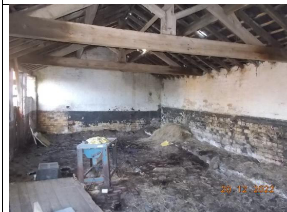
Plate 8: Building 2, showing the former livestock stall.
