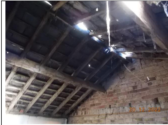
Plate 6: Building A, showing the roof and the internal timber frame.
