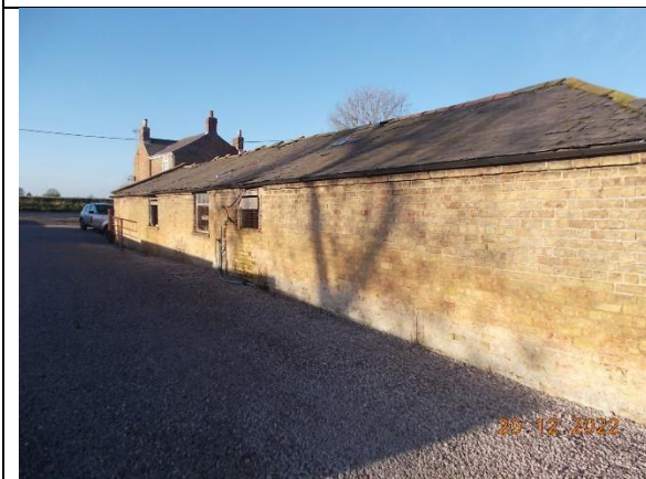
Plate 2: Building A. Photograph taken from the south-east.
