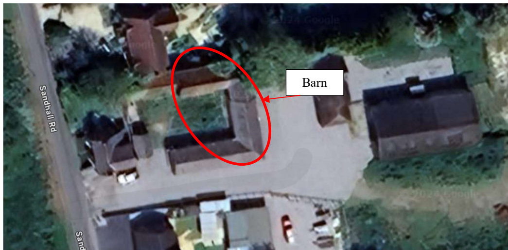
Aerial View of Barns
