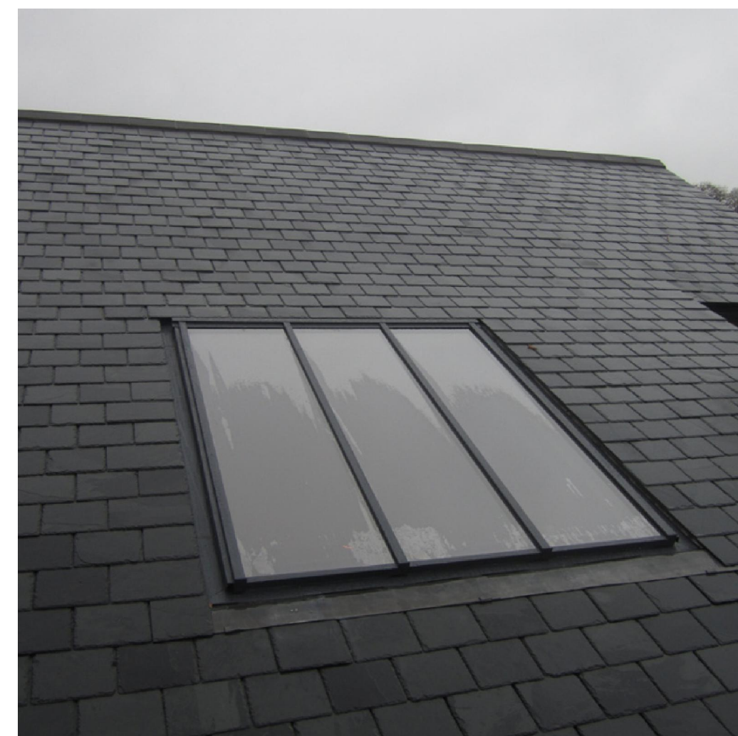
Patent Roof Glazing Example
