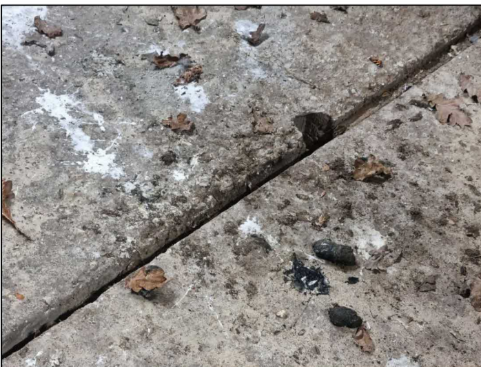
f) Barn owl pellets below rafter in stables.
