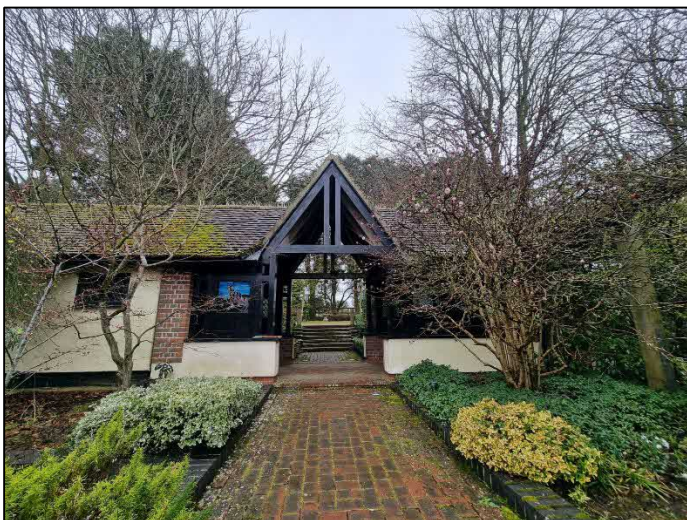
c) Log store/porch building, to be extended to the west.
