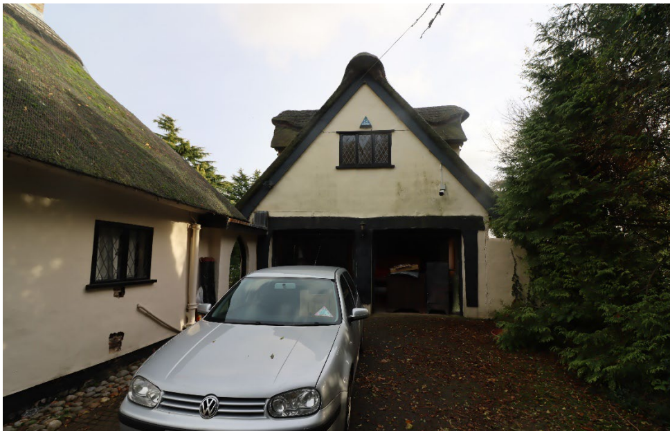
Figure 3. North East Gable Elevation of South West Cottage. Garage doors to be infilled leaving two sets of casement flush timber windows at ground floor. Chimney stack formed towards right side.
