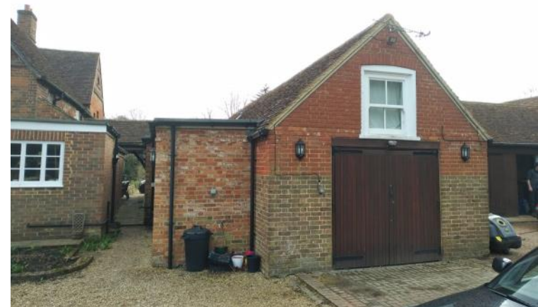
Figure 5.75: Showing the northern elevation of the Western Annex.
