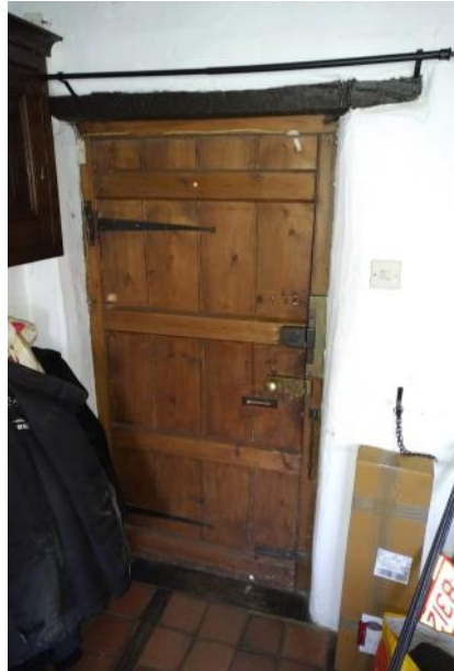
Figure 5.80: Showing the door from the Breakfast Room to the covered walkway.
