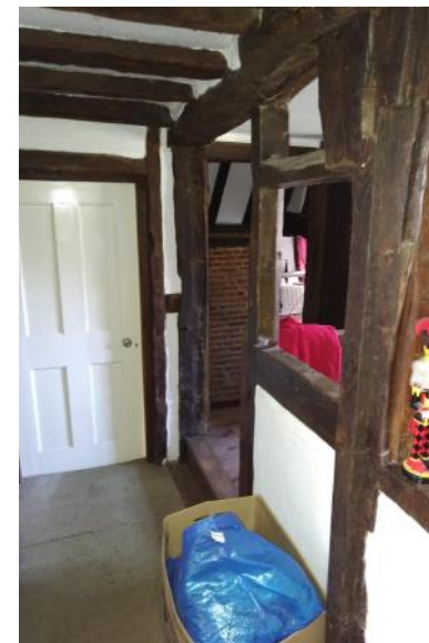
Figure 5.145: Showing the 17th century former mullioned window to the landing opposite the Mid C20 Staircase.
