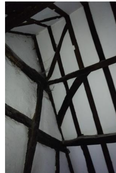
Figure 5.193: Showing the curved wind braces at the southern end of the room.
