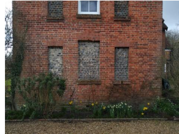
Figure 5.36: Showing the ground floor of the Front Range's eastern elevation.
