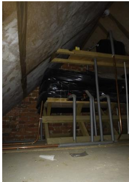
Figure 5.157: Showing the plasterboard ceiling to the bathroom.
