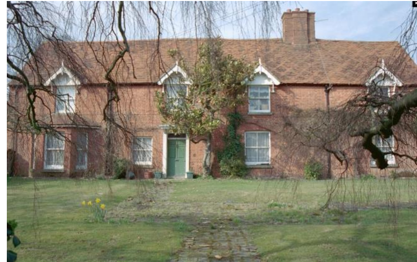
Figure 5.9: Front elevation in 2003 (Source: Historic England list entry).
