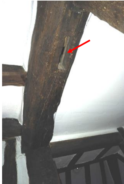
Figure 5.147: Showing the doorway opening from the Rear Corridor allowing access to the Master Bedroom. The mortise joint for the former post in this location is marked in red.
