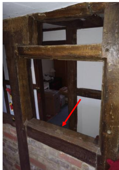
Figure 5.145: Showing the 17th century former mullioned window to the landing opposite the Mid C20 Staircase.
