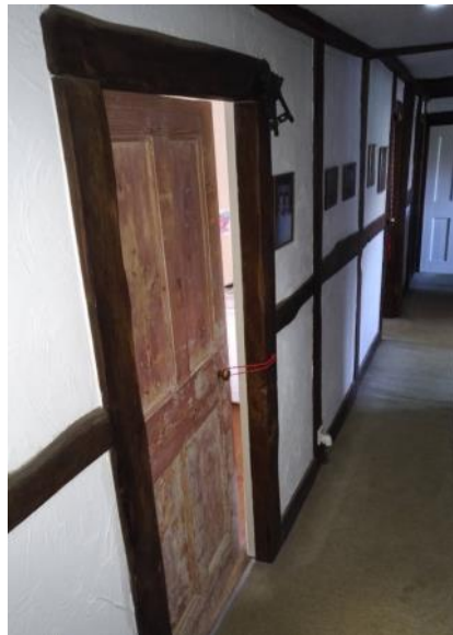
Figure 5.149: Showing the southern side of the Rear Corridor. All timber framing shown is modern except the historic elements shown at Figure 5.148.
