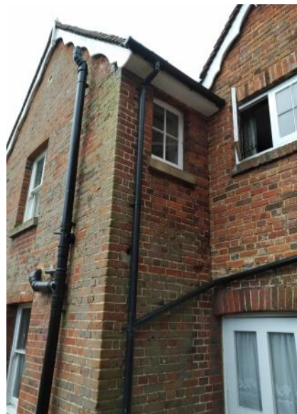
Figure 5.49: Showing the western elevation of the Victorian Extension.
