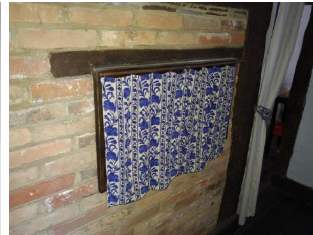
Figure 5.130: Showing the service hatch in the Rear Corridor.
