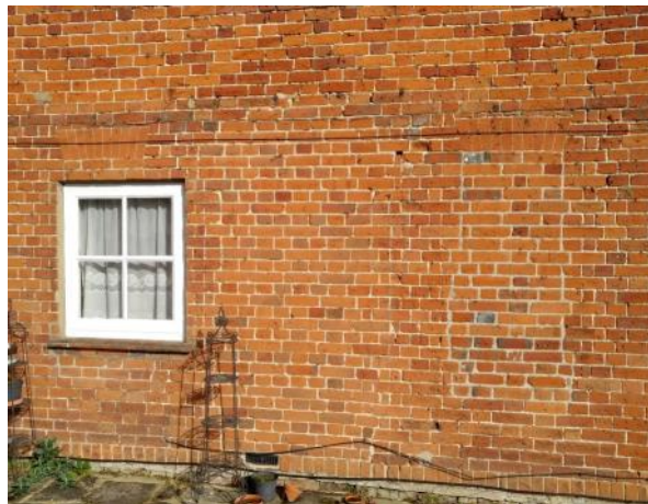
Figure 5.33: Showing the ground floor of the Front Range's western elevation.
