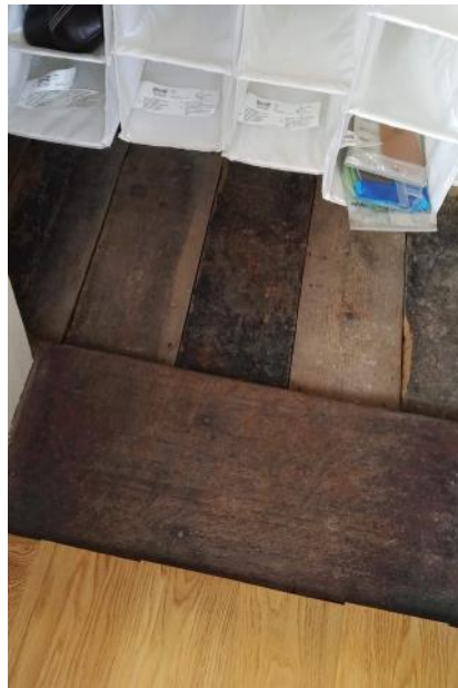
Figure 5.183: Showing the historic floorboards within the Western Bedroom's cupboard.
