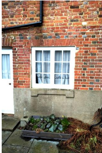
Figure 5.51: Showing the ground floor window to the former outshut.
