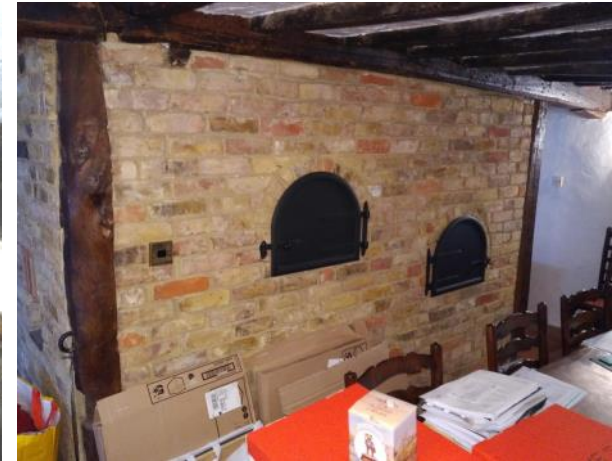
Figure 5.89: Showing the bread ovens to the southern side of the Dining Room on the fireplace's rear wall.
