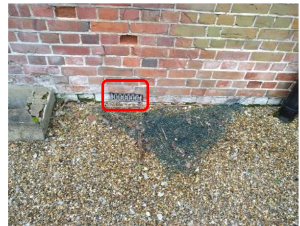
Figure 5.50: Showing the airbrick to the base of the Victorian Extension.
