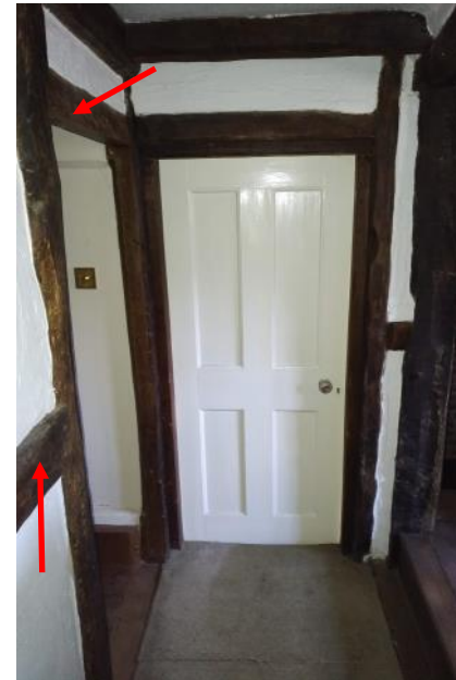
Figure 5.147: Showing the doorway opening from the Rear Corridor allowing access to the Master Bedroom. The mortise joint for the former post in this location is marked in red.
