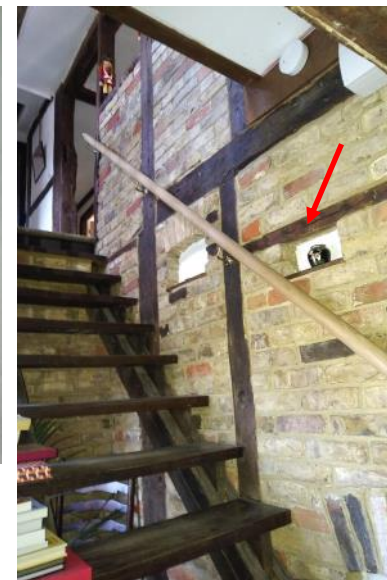
Figure 5.141: Showing the RSJ between the Mid C20 Staircase and the Dining Room.
