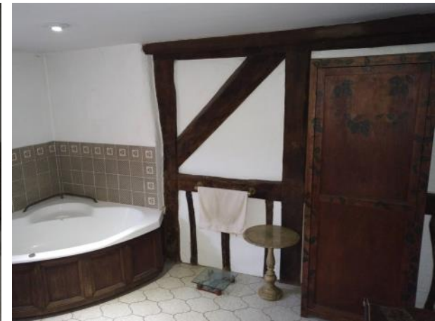
Figure 5.154: Showing the eastern wall of the bathroom and a 17th century straight brace from the earlier 17th century stair core.
