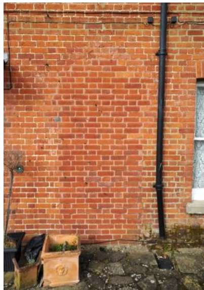
Figure 5.25: Showing the former location of the former central entrance, since infilled. Note the brickwork is a slightly darker hue.
