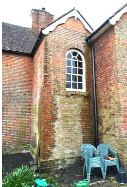
Figure 5.43: Showing the Georgian stair core.
