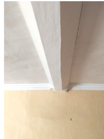
Figure 5.170: Showing the ceiling's central beam.
