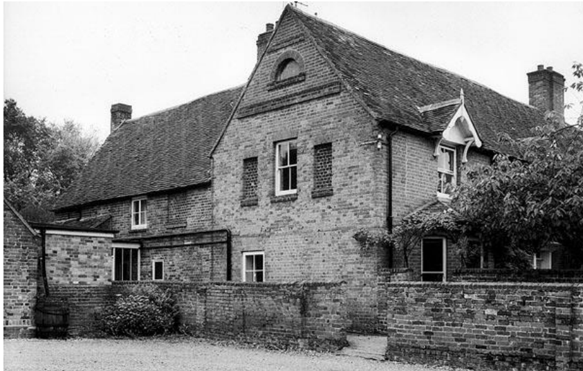
Figure 5.8: View showing the house's western end in 1972. Note the diapered roof tiling to the Rear Range (Source: Surrey Archives).
