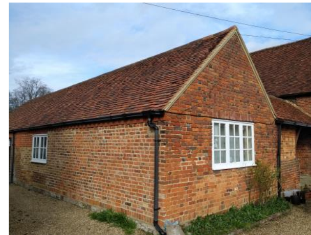
Figure 5.73: Showing the southern and western elevations of the Western Annex.
