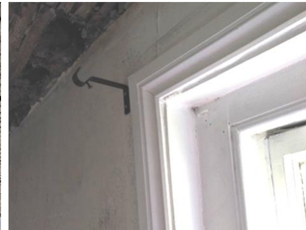
Figure 5.134: Showing the modern architrave to the W.C. ante-room window.
