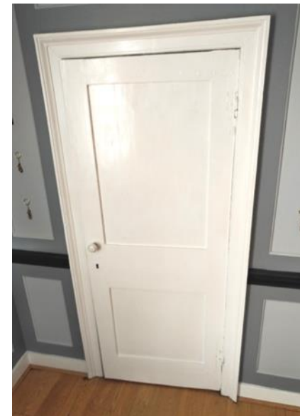
Figure 5.182: Showing the cupboard door and architrave in the Western Bedroom.
