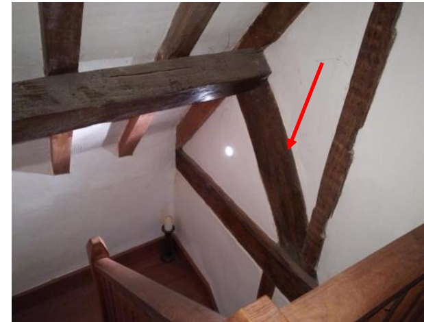
Figure 5.199: Showing the 17th century curved brace forming part of the timber framing exposed in the creation of the new loft stairwell.
