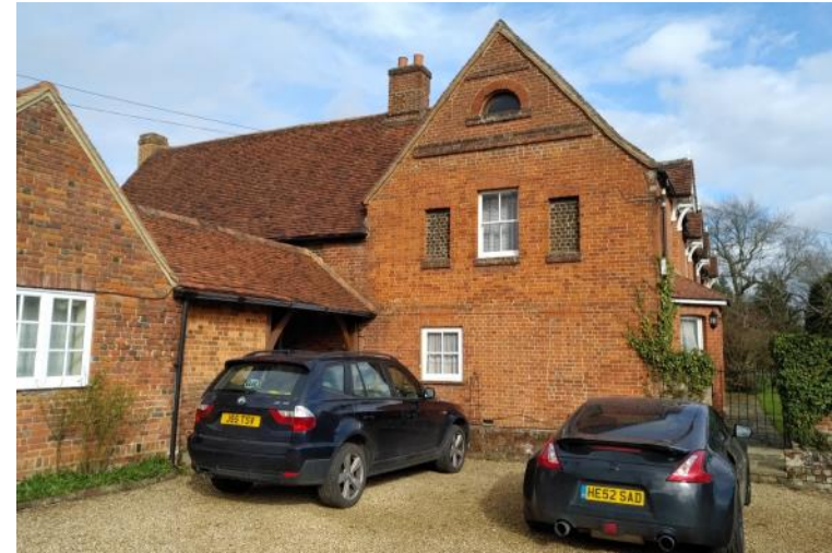
Figure 5.74: Showing the southern elevation of the covered walkway.
