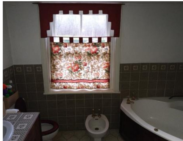
Figure 5.153: Showing the northern wall of the bathroom and its original window architrave.
