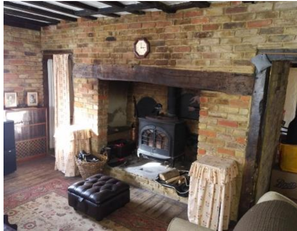
Figure 5.92: Showing the largely rebuilt fireplace on the northern side of the Sitting Room.
