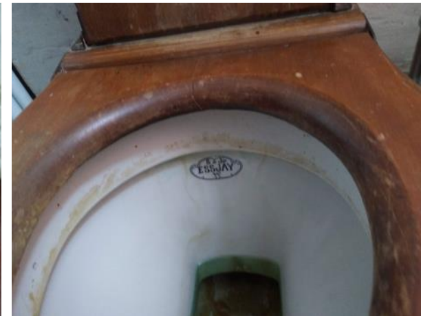
Figure 5.138: Showing the W.C..
