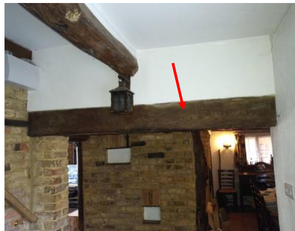
Figure 5.141: Showing the RSJ between the Mid C20 Staircase and the Dining Room.
