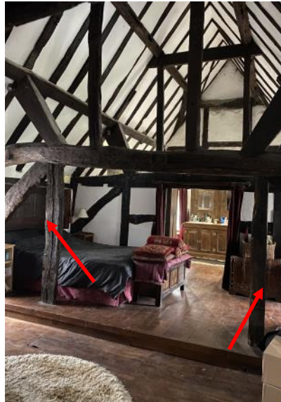
Figure 5.187: Showing the Master Bedroom as seen from the entrance doorway. The two modern posts added by the present owners are marked in red.
