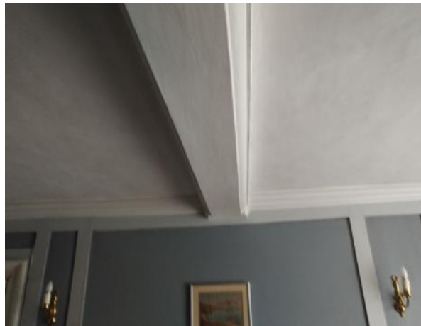
Figure 5.103: Showing the chamfered central ceiling beam to the Music Room.
