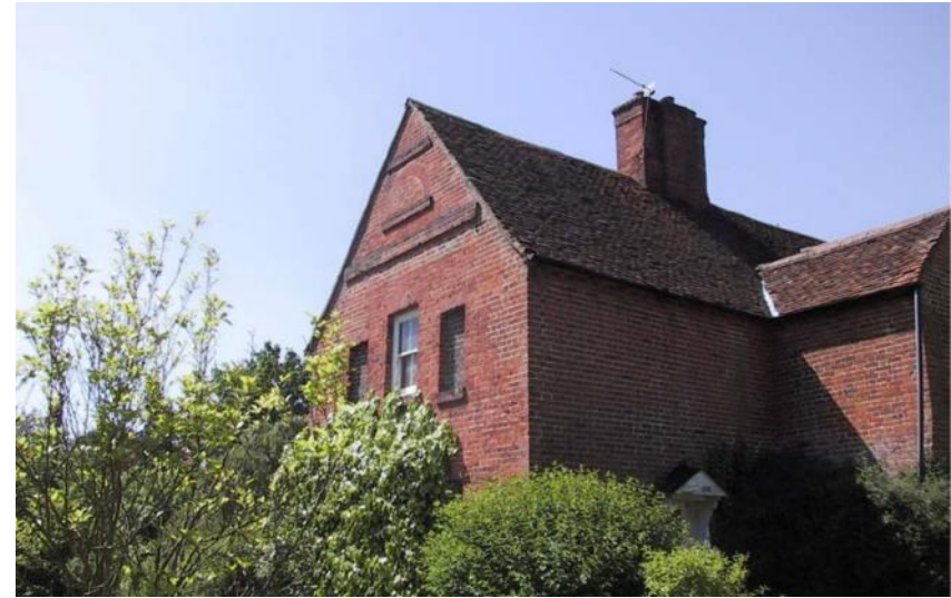
Figure 5.13: View showing the Front Range's eastern elevation (first floor) in 2004 (Source: Phillip Arnold).
