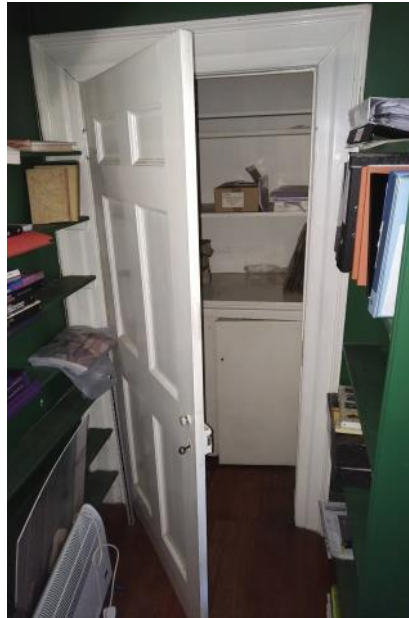
Figure 5.123: Showing the cupboard door and architrave to the Office.
