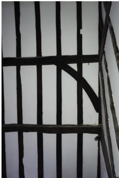
Figure 5.193: Showing the curved wind braces at the southern end of the room.
