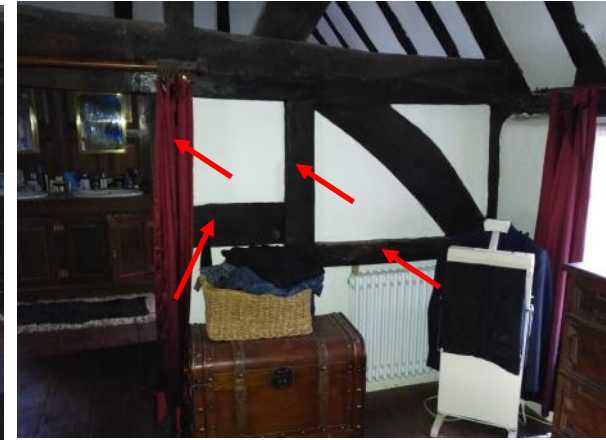
Figure 5.192: Showing the middle bay of the room (eastern side). The timber members added by the present owners are marked in red.
