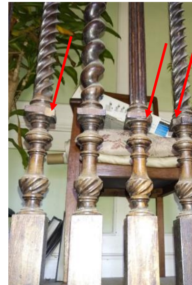
Figure 5.121: Showing the balustrade to the first floor staircase landing where it has become loose from the wall (marked in red).
