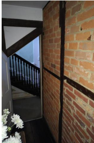
Figure 5.127: Showing the brickwork to the infill panel closest to the Main Staircase.
