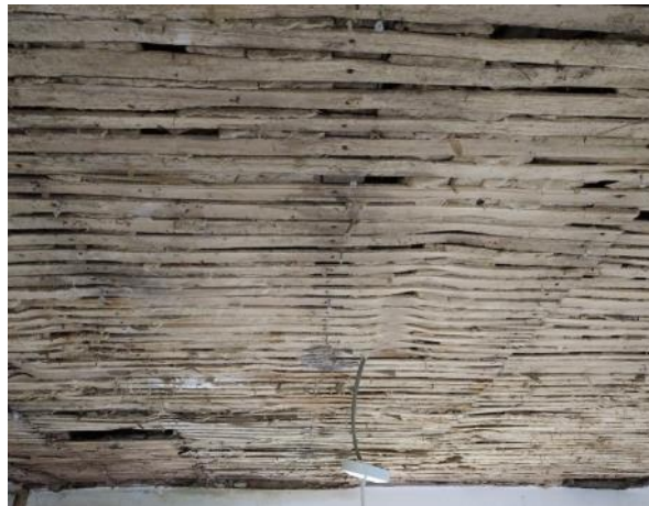
Figure 5.133: Showing the lath and plaster ceiling to the W.C. ante-room.
