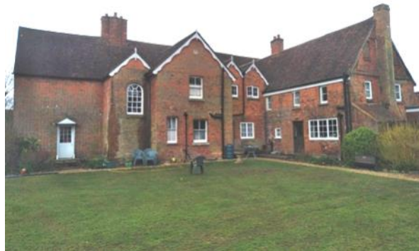
Figure 5.41: Showing the rear elevation of the Front Range and the eastern elevation of the Rear Range.
