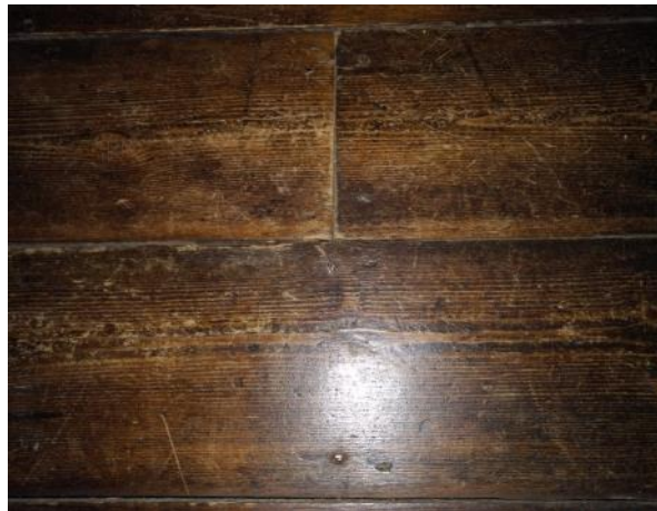
Figure 5.94: Showing the boarded floor to the Sitting Room.
