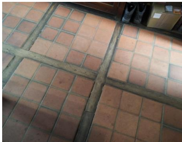
Figure 5.82: Showing the oak framed floor inset with red clay quarry tiles.
