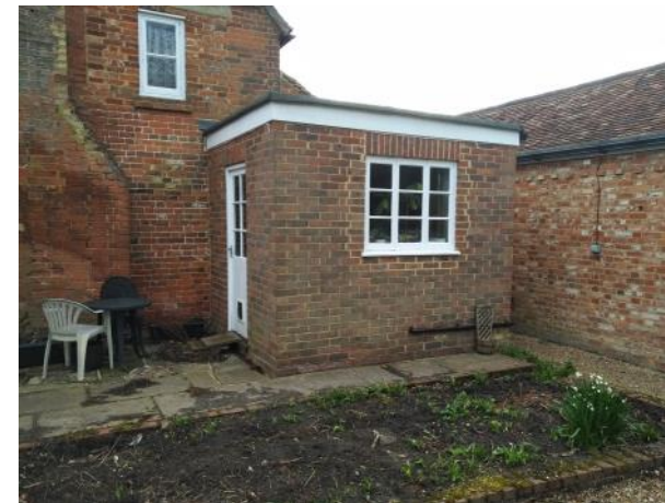
Figure 5.65: Showing the northern elevation to the 1960s extension.
