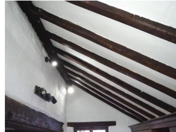
Figure 5.77: Showing the monopitched roof above the Kitchen.
