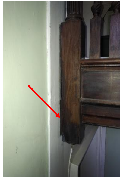
Figure 5.121: Showing the balustrade to the first floor staircase landing where it has become loose from the wall (marked in red).
