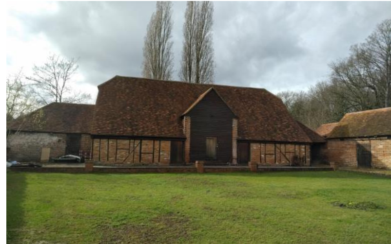
Figure 6.10: Listed barn near house.
