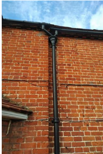
Figure 5.27: Showing how the front elevation is slightly steeped forward to its western and eastern ends. Also note the uPVC guttering and the cables attached to the brickwork.
