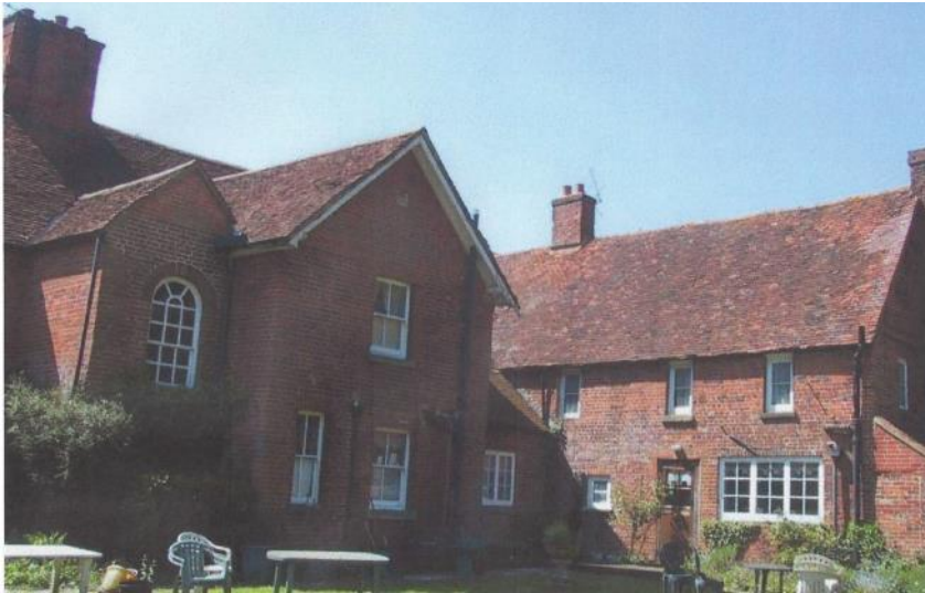
Figure 5.12: Showing part of the Front Range's rear elevation and the eastern elevation of the Rear Range in 2004 (Source: Phillip Arnold).
