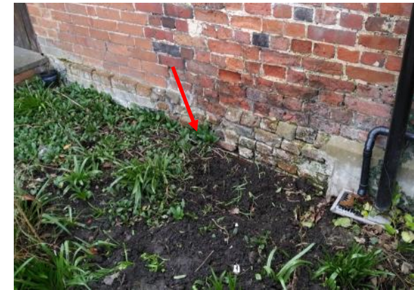
Figure 5.59: Showing the brick plinth to the original timber framed building.
