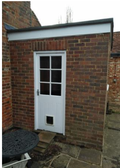
Figure 5.64: Showing the eastern elevation to the 1960s extension.
