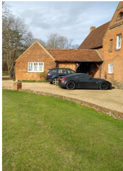
Figure 5.72: Showing the southern elevation of the Western Annex and the covered walkway.
