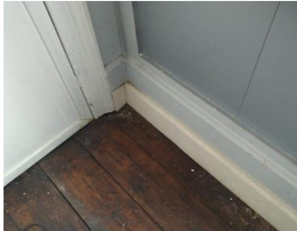
Figure 5.105: Showing a section of double skirting boards on the southern wall of the Music Room.
