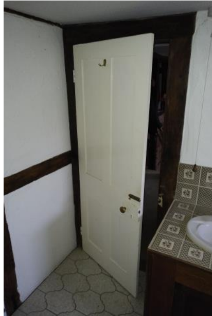
Figure 5.155: Showing the 4-panelled door to the bathroom.
