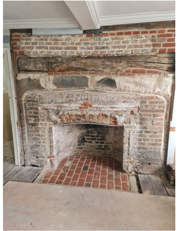
P.35 - Music Room - SE Elevation Repairs to fireplace and hearth
