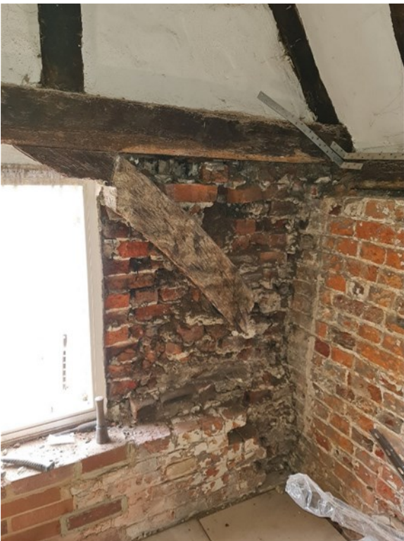
P.48 - 1st Floor Master En-suite - N/NE Corner
