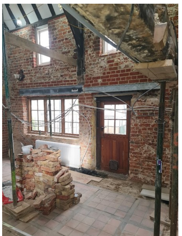
P.22 - GF - NE Elevation Replacement of rotten Lintels
