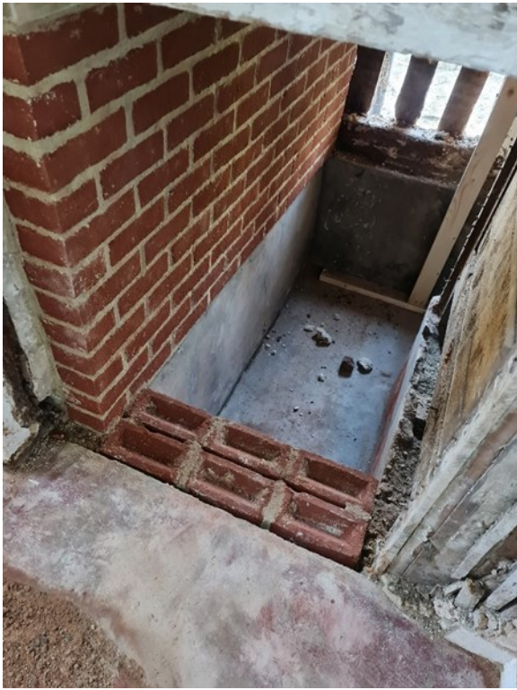
P.38 - GF Basement to Stair Landing - NE Elevation New skin of brickwork taken up to support stair landing, and new 1 brick thick retaining wall to toilet floor
