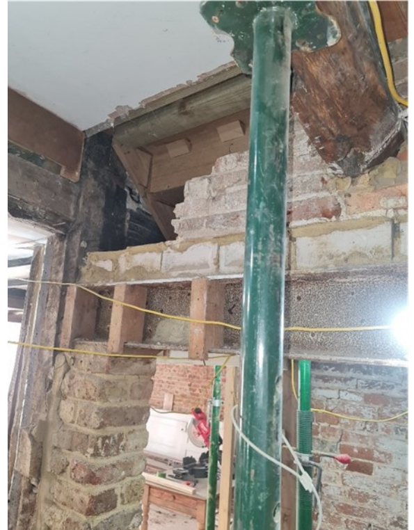
P.18 - GF Stairwell
