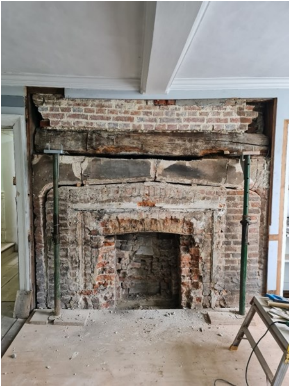
P.34 - GF Music Room - SE Elevation Repair process underway
