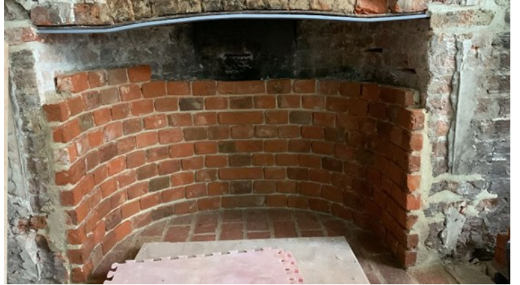
P.37 - Music Room - SE Elevation Rebuilding of hearth & fireplace chimney brickwork
