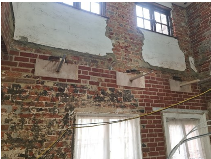
P. 25 - GF - NE Elevation - Stairwell
