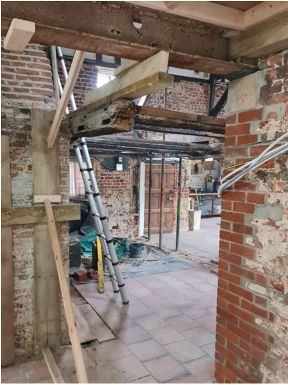
P. 26 - GF Stairwell & Dining Room
