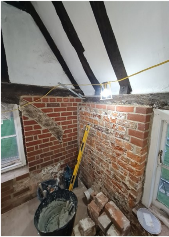
P.50 - 1st Floor Master En-Suit - NE Corner Brickwork reconstruction Note 20 - DRWG CLT Ltd - P101
