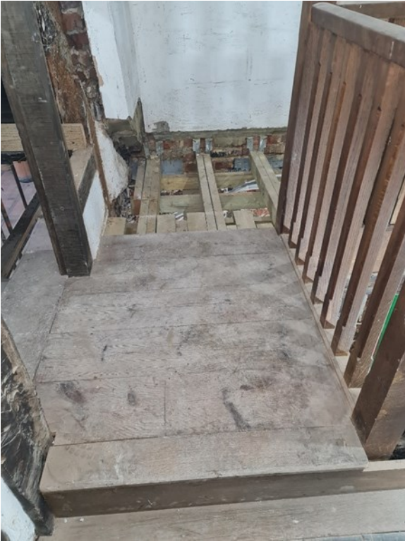
P.46 - 2nd Floor - Stairwell Landing
