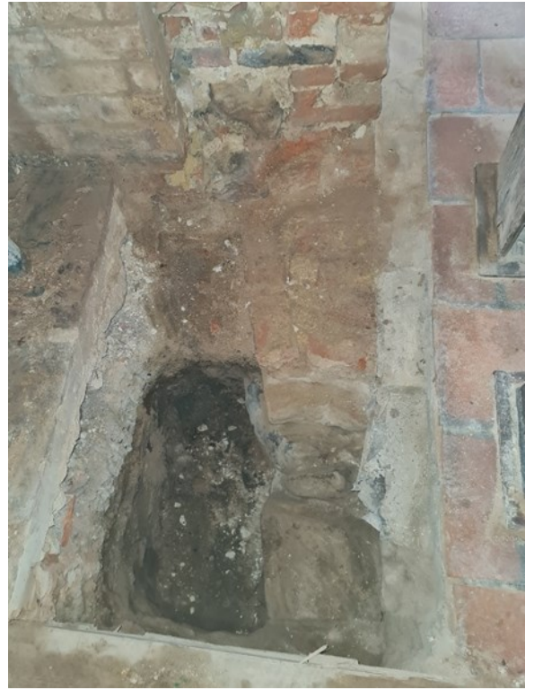
P.16 - GF Lounge / Stairwell
