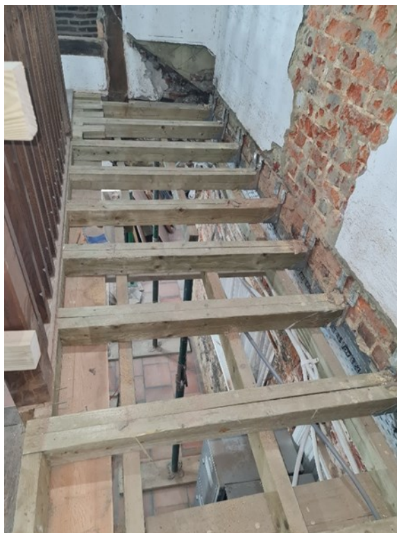
P.45 - 1st Floor - Stairwell Landing
