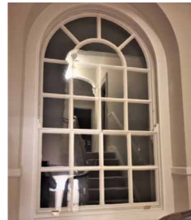
Fig 42. Example image of secondary glazing on existing sash window. Supplied by Mitchell & Dickinson
