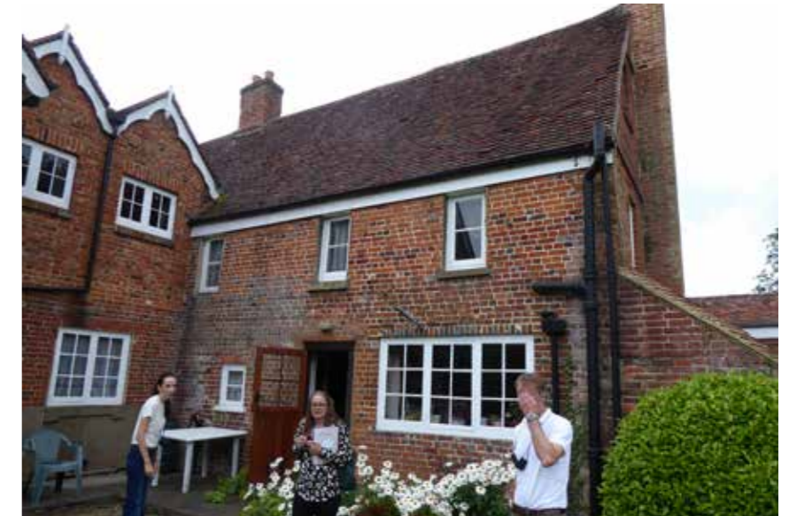
Fig. 25 Evidence of multiple approaches to window cill detailing on rear elevation. Timber, concrete and bricks cills are shown in this image.
