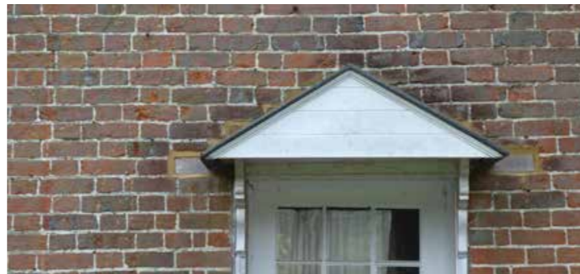
Fig. 23 Mid-20 th Century painted timber canopy over rear door.
