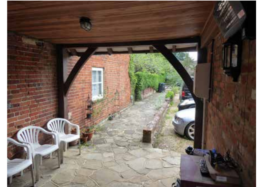
Fig 33: Concrete external paving.
