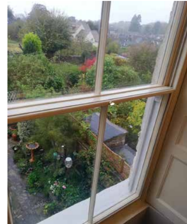
Fig 41. Example image of secondary glazing on existing sash window. Supplied by Mitchell & Dickinson
