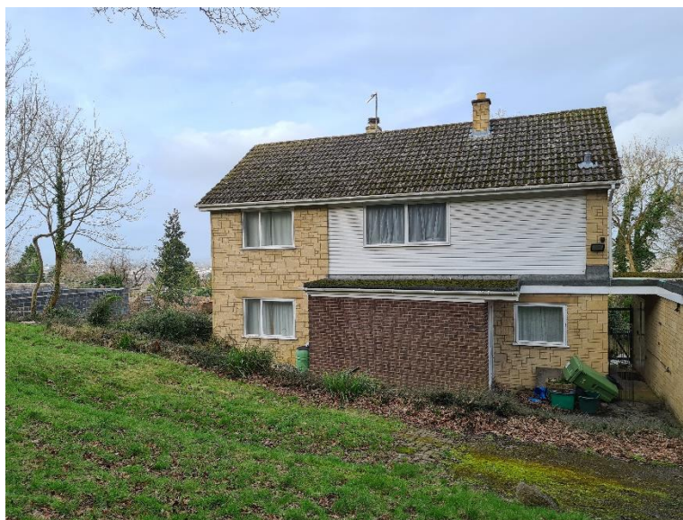
View of the existing property viewed from access drive
