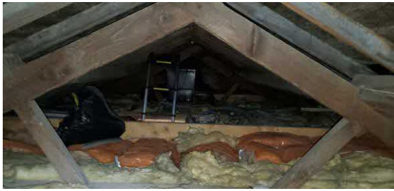
9 Internal view of northern loft void
