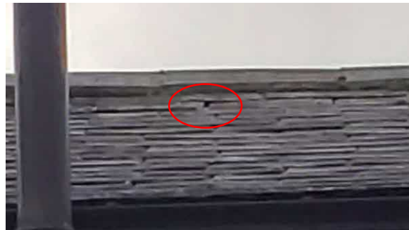
6 Gap between slates
