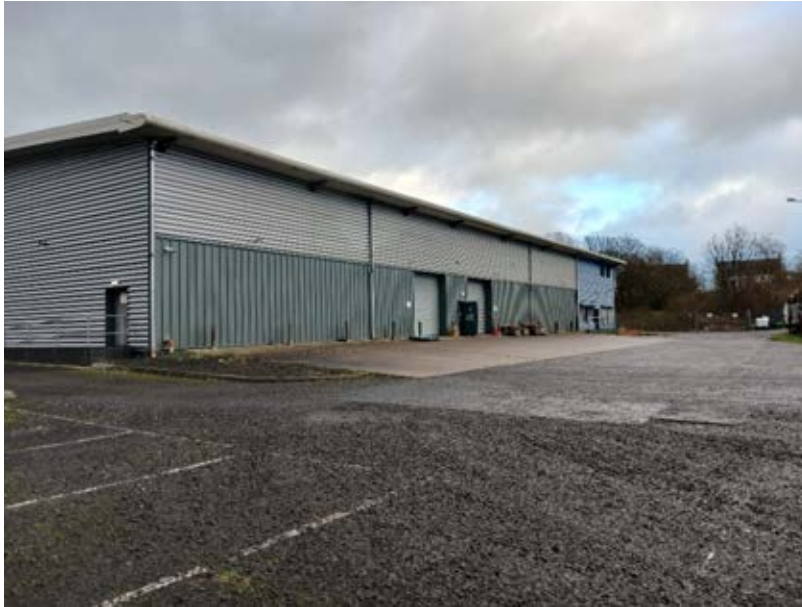
Photograph 1 – Southern face of warehouse and area where extension is proposed. Taken facing NE.
