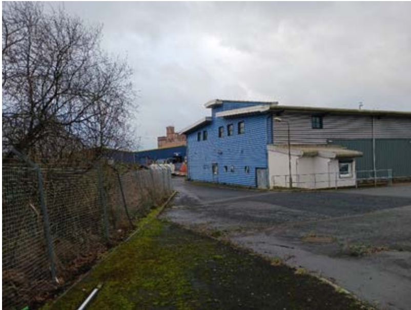
Photograph 4 – Eastern face of warehouse and eastern boundary. Photo taken facing S/SW.
