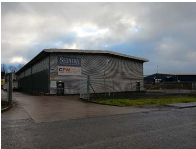
Photograph 18 – Northern-most entrance gate into the site. Photo taken from Denburn Road, facing E towards site.
