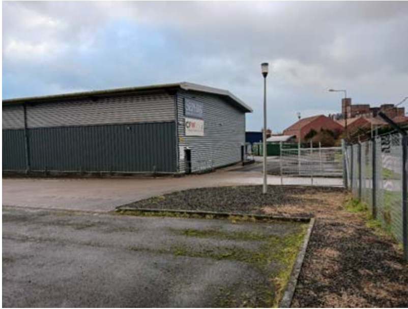
Photograph 3 – Western face of warehouse and western boundary. Photo taken facing S/SE.
