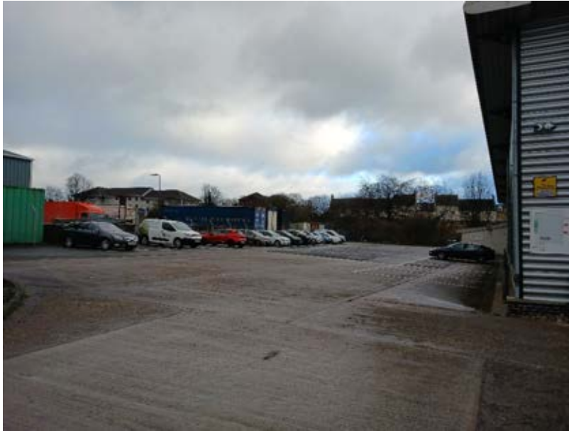
Photograph 5 – Carpark area to north of warehouse. Photo taken facing NE.
