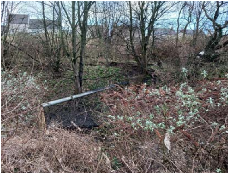
Photograph 14 – Burn to east (outwith site perimeter), before it becomes culverted; culvert appears to go beneath site protrusion in east. Pipe above burn enters eastern boundary of site. Photo taken facing E from eastern boundary.
