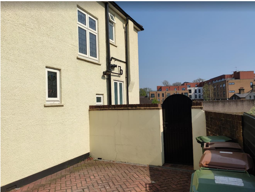
Figure 4: Photo of the southern side of the property at ground floor level
