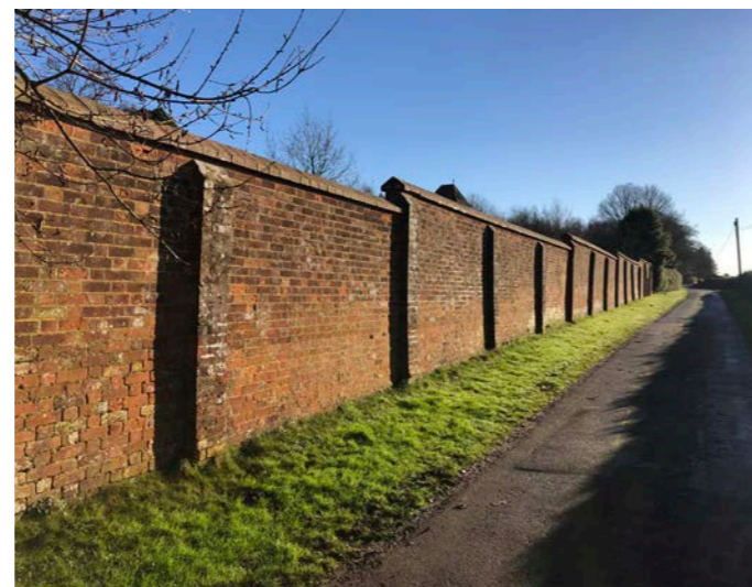
1 Historic Brick Wall on Southern Boundary
