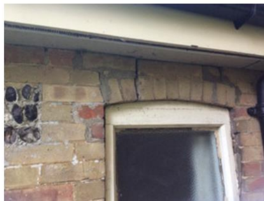
Picture 3: External cracking to right elevation Picture 4: External cracking to right elevation
