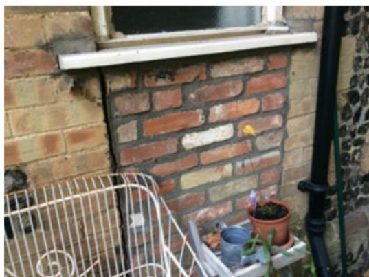
Picture 3: External cracking to right elevation Picture 4: External cracking to right elevation
