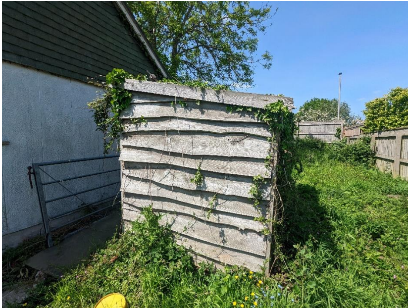
Figure 4.6. Shed at the northern extent
