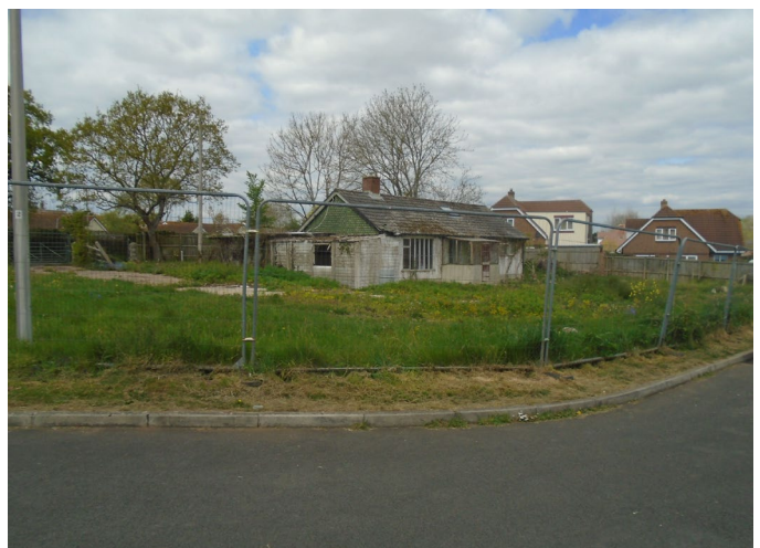
Image: View of existing dwelling from Whitecross Gardens
